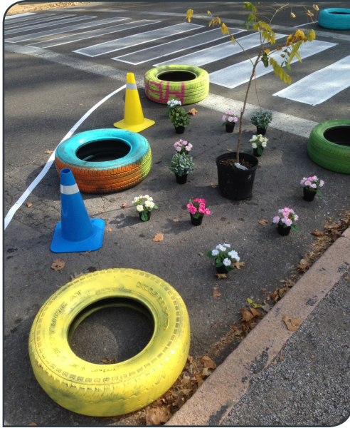
The traffic cones, plants, and colorfully painted tires are arranged as a curb extension, which narrows the road in order to slow traffic and shortens the crossing distance for people walking. Photo: TrailNet
