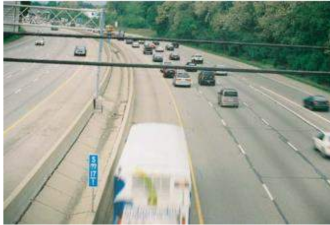
Figure 2-4: I-71 Left Shoulder Bus-on-Shoulder
