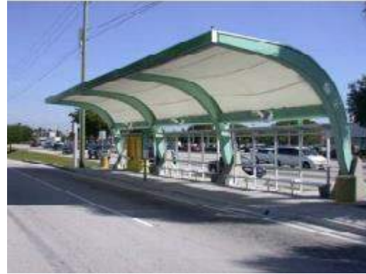
Figure 2-6: South Dade Busway Station
