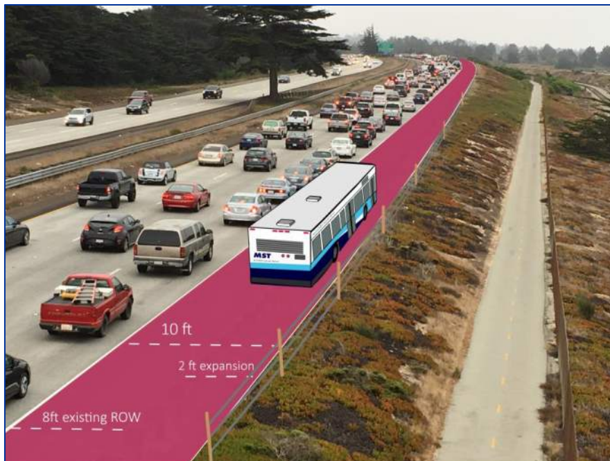
Figure 1-6 - Depiction of Bus-on-Shoulder on SR-1 Southbound
