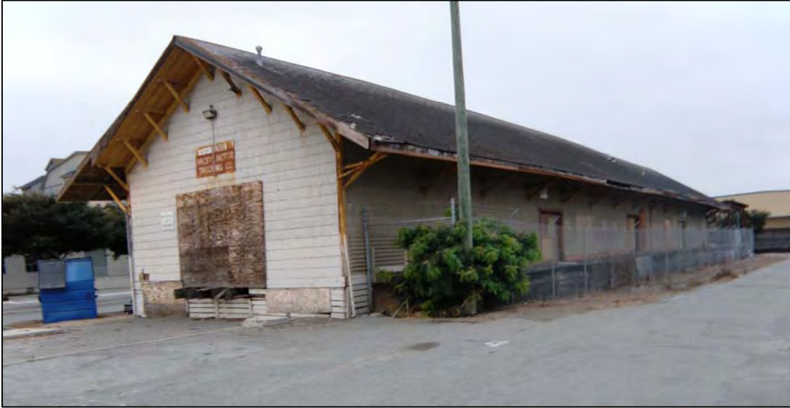
Depot, south and northeast façades, view to west. Photograph taken October 16, 2010.
