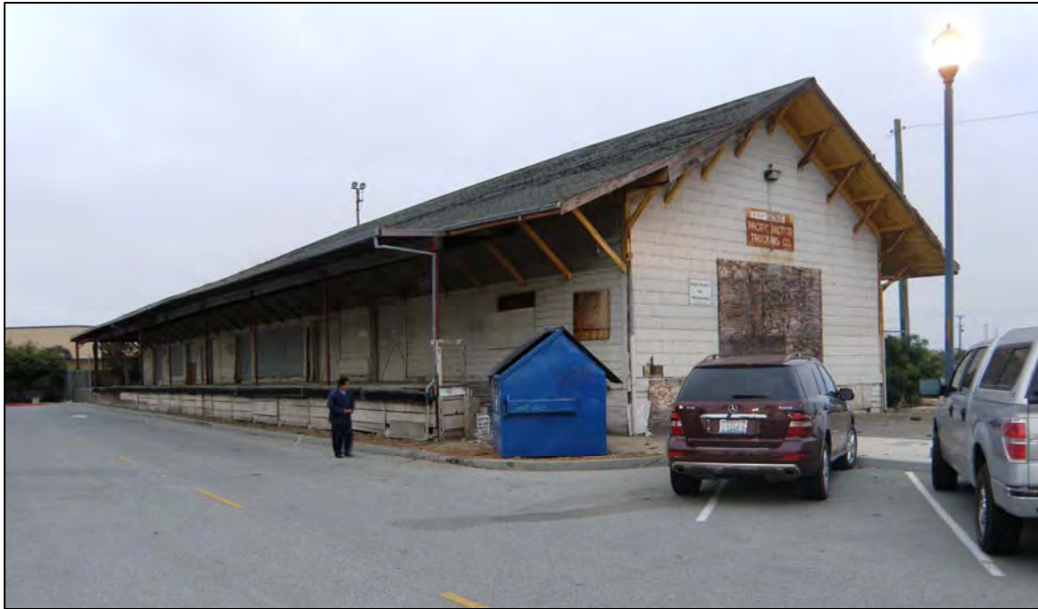
Depot Building, southwest and southeast façades, view to north. Photograph taken October 16, 2010.
