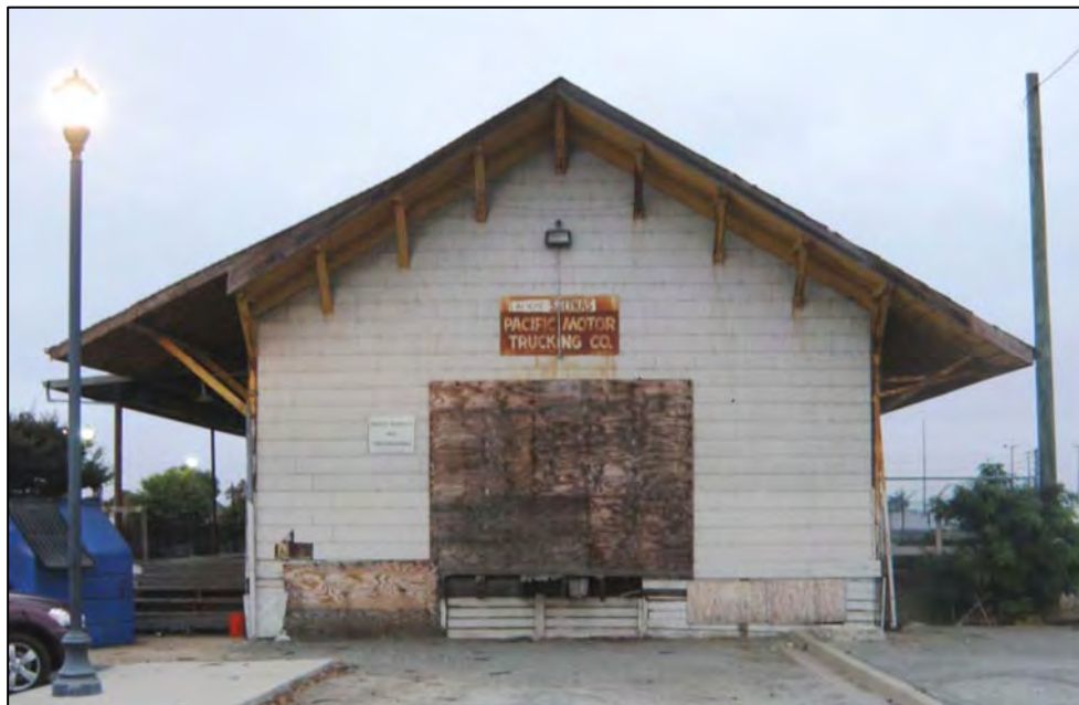
Depot Building, south façade, view to northwest. Photograph taken October 16, 2010.
