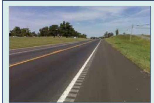
EDGE-LINE RUMBLE STRIP
