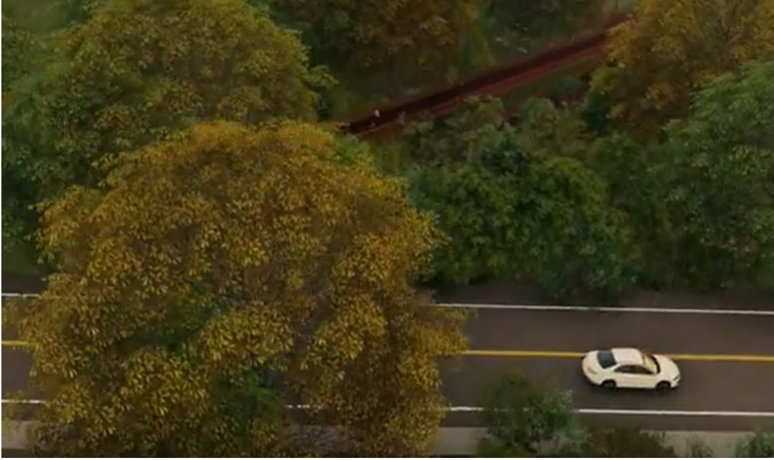
Looking east toward the Frog Pond Wetland Preserve and raised pathway across Canyon Del Rey/SR 218.
