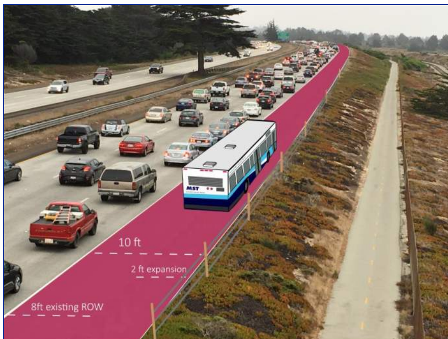
Figure 1-6 - Depiction of Bus-on-Shoulder on SR-1 Southbound
