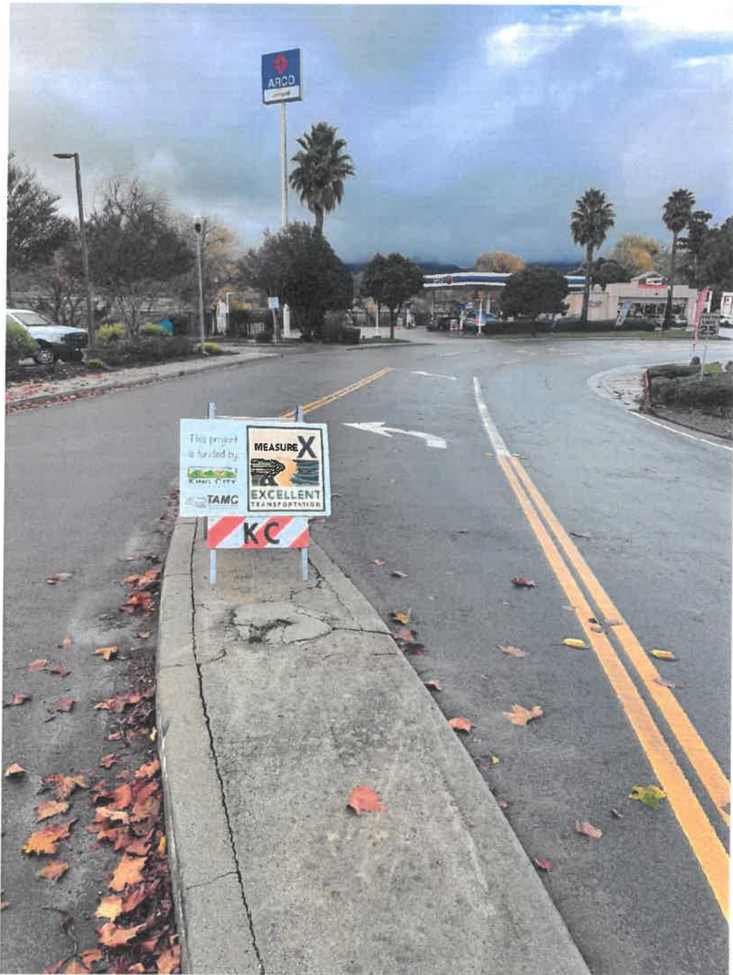
Figure 2 Broadway Street - After Construction
