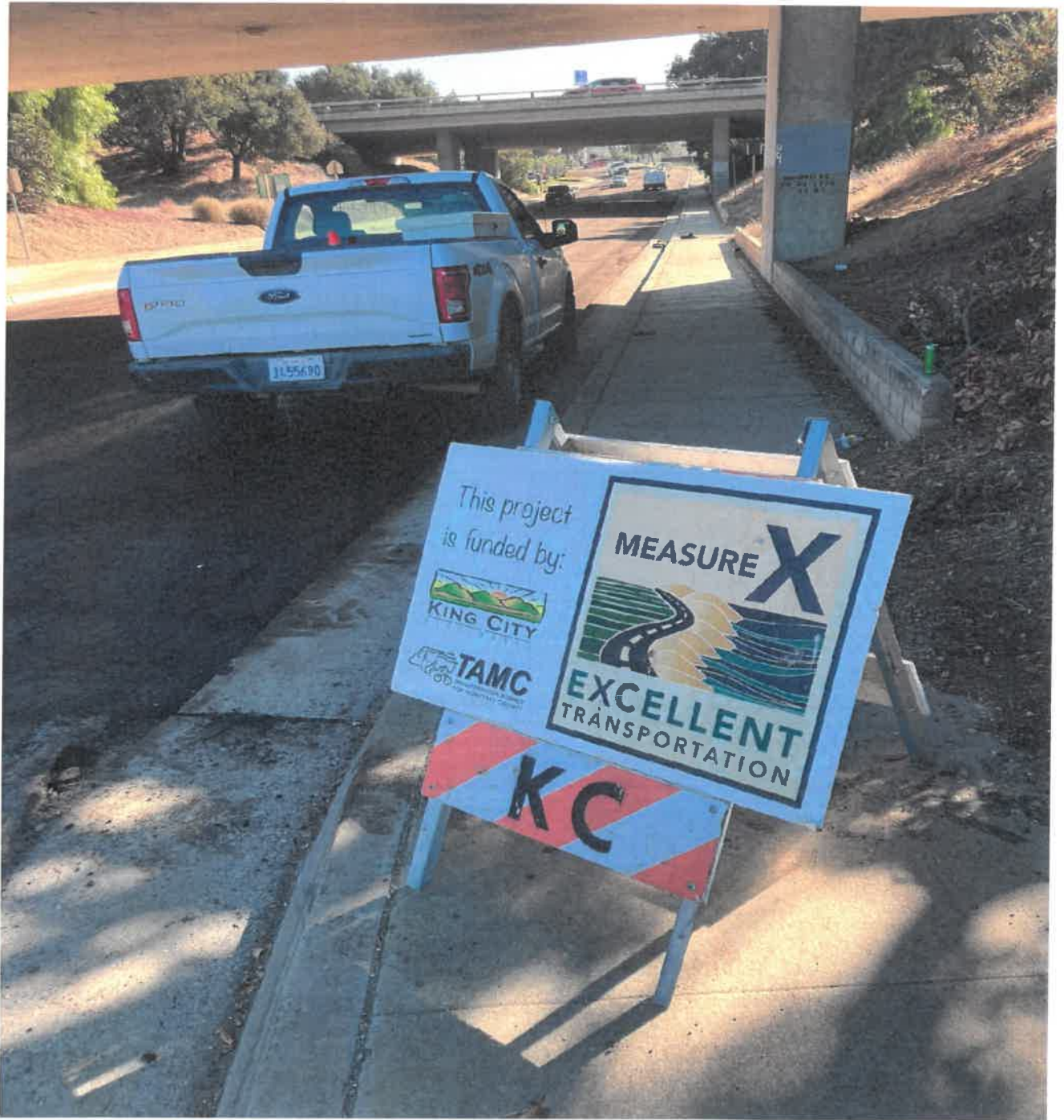
Figure 1 Broadway Street - During Construction
