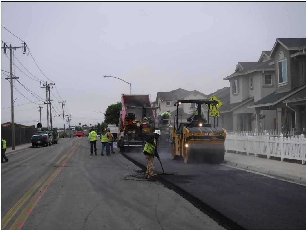
Placing hot-mix-asphalt
