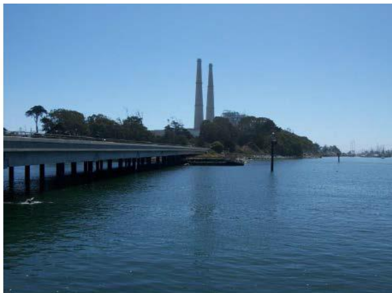
North end of project looking south toward Moss Landing Harbor. The Elkhorn Slough Bike Bridge will span Elkhorn Slough parallel to the existing State Route 1 Bridge. The Elkhorn Slough Bike Bridge will include rest area to stop and enjoy the scenery.
