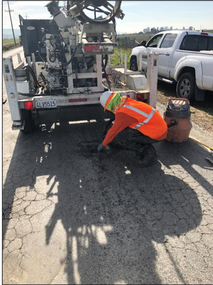
Coring on Old Stage Road
