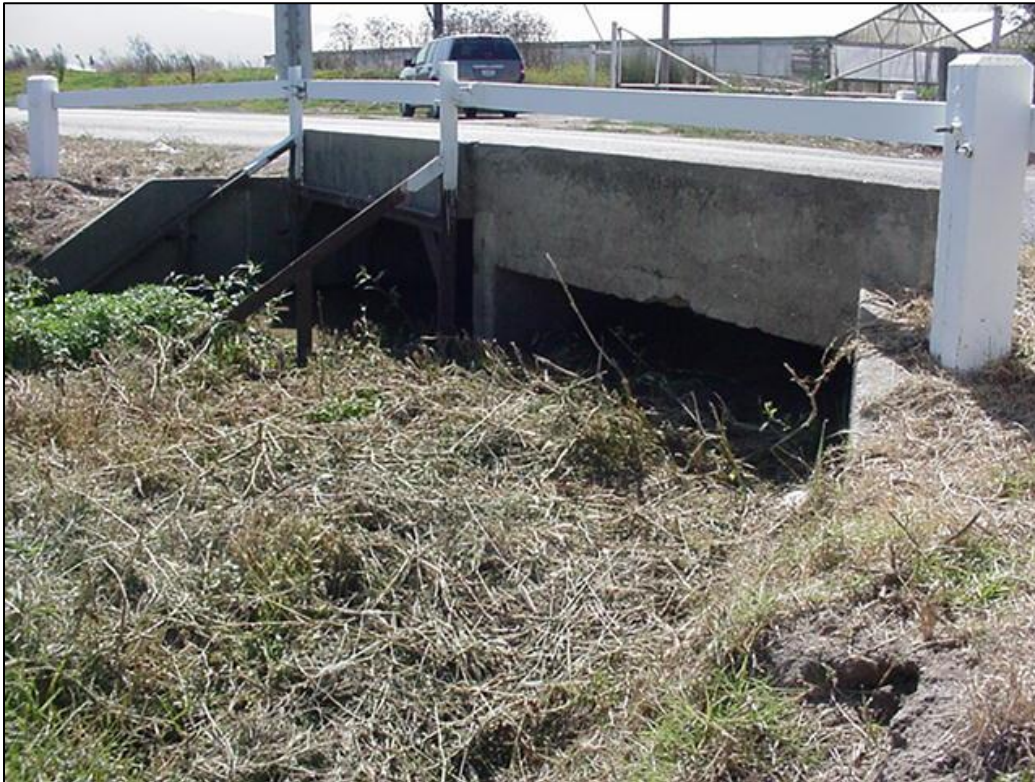
Hartnell Road Bridge
