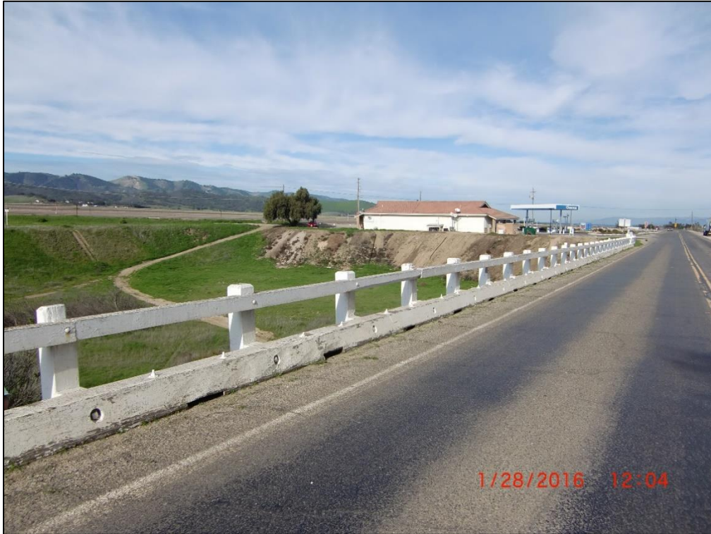
Existing Rail on Jolon Rd Bridge
