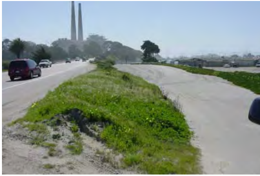
An existing easement through the Duke Energy Plant along Highway 1 presents an opportunity for trail alignment.
