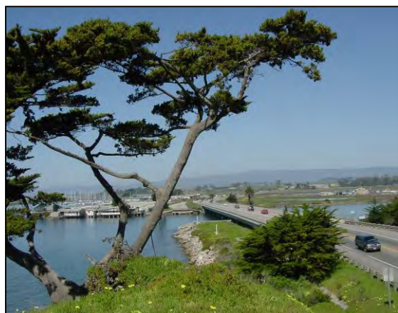
Looking north at the Moss Landing Bridge
