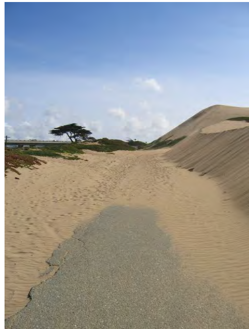
Sand can render trail facilities unusable. Design measures should be taken to counteract the sand and regular maintenance should be performed.
