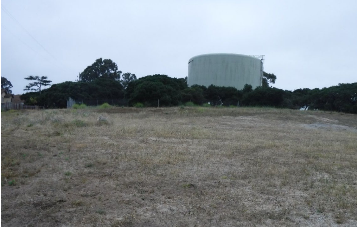
Photograph 33. 6.20.2019. Water tower located along the Northern Loop Trail segment with annual grassland in the foreground, facing west.
