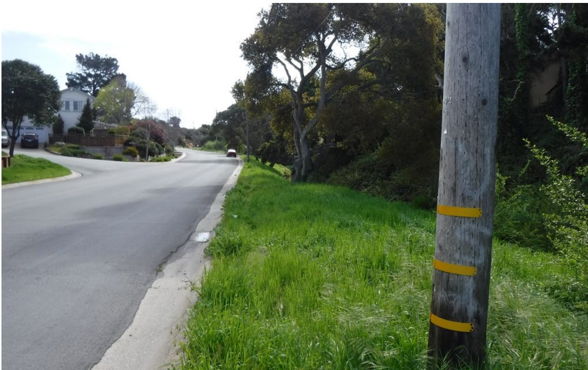
Photograph 6. 3.28.2019. The Canyon Del Rey/ SR 218 Trail segment at Angelus Way, Canyon Del Rey Creek can be seen to the left of the road, facing east.
