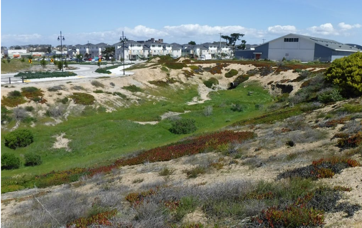
Photograph 23. 3.29.2019. A detention basin with iceplant mat at west end of the CSUMB north Loop Trail segment, facing north east.
