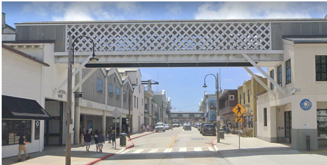
Before Rectangular Rapid Flashing Beacon Installed, 2019
