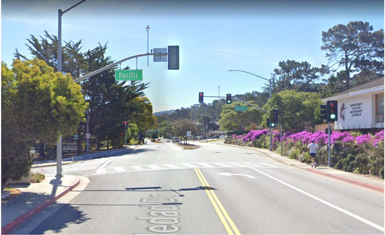
After Protected Left Turns Installed Soledad Dr at Pacific St
