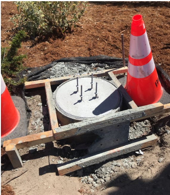
Wayfinding sign foundation construction
