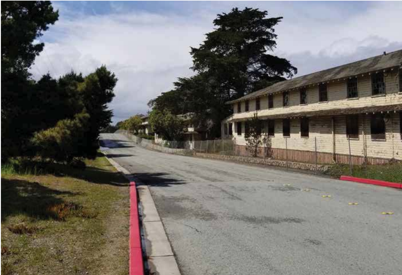
Example of vacant barracks found throughout this segment
