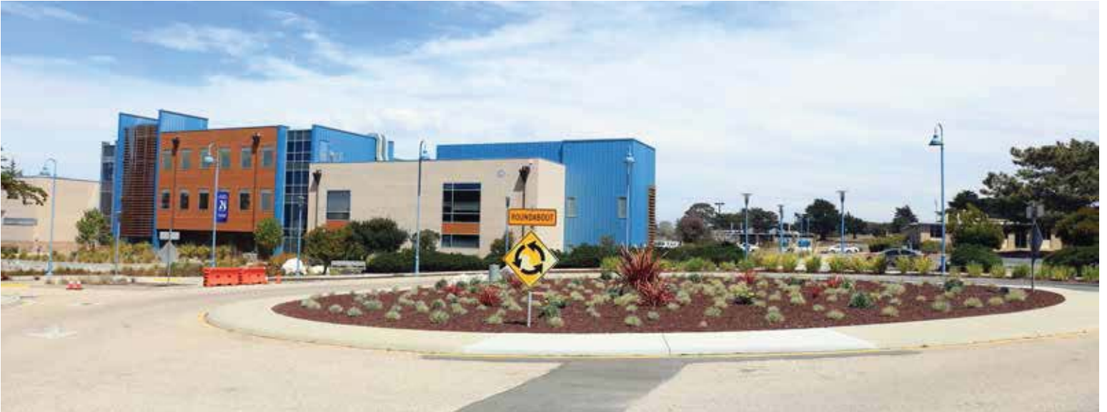
Example images of existing context found along the CSUMB Loop South Segment
