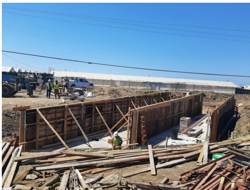
Form work for new bridge
