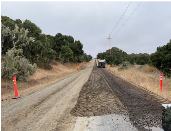
Full-depth reclamation process
