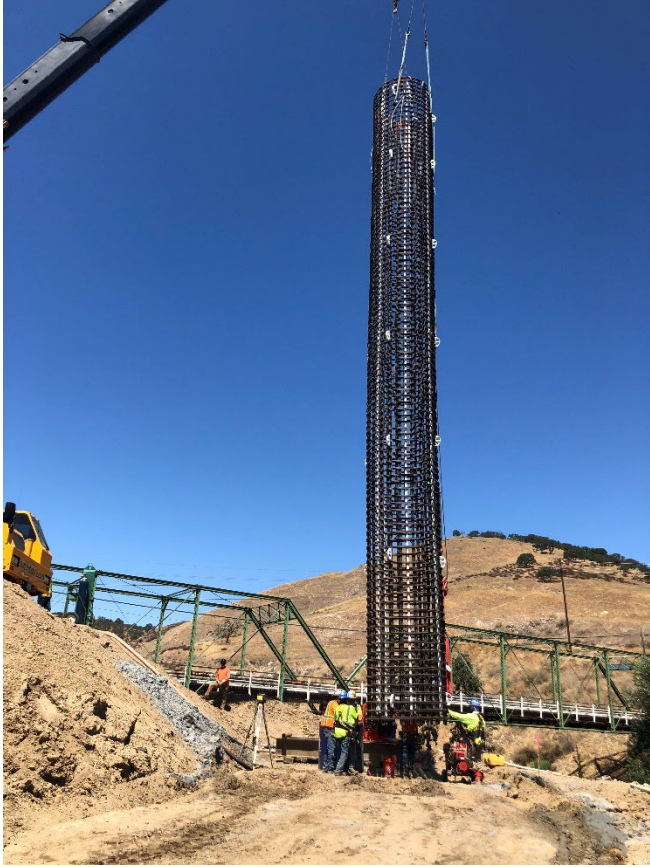
Setting of rebar cage for pier
