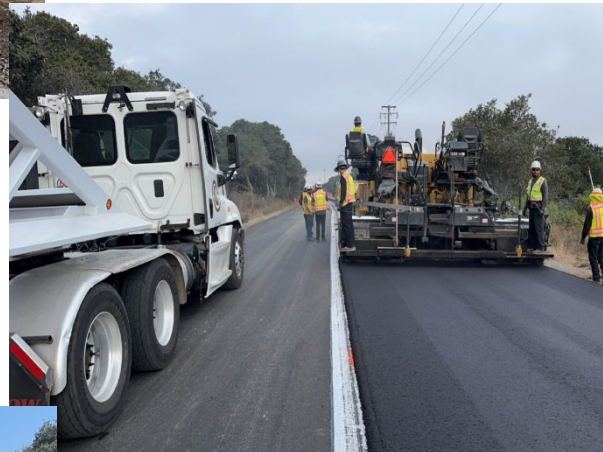
Placing Asphalt Concrete
