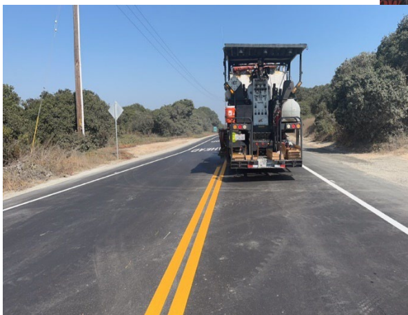
Placing Pavement Traffic Stripes
