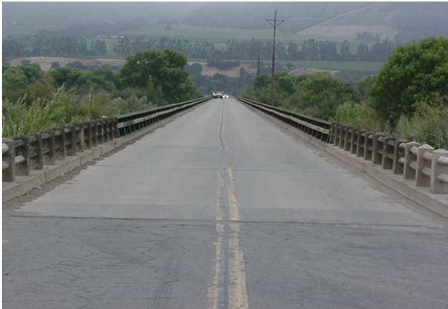
Existing bridge superstructure
