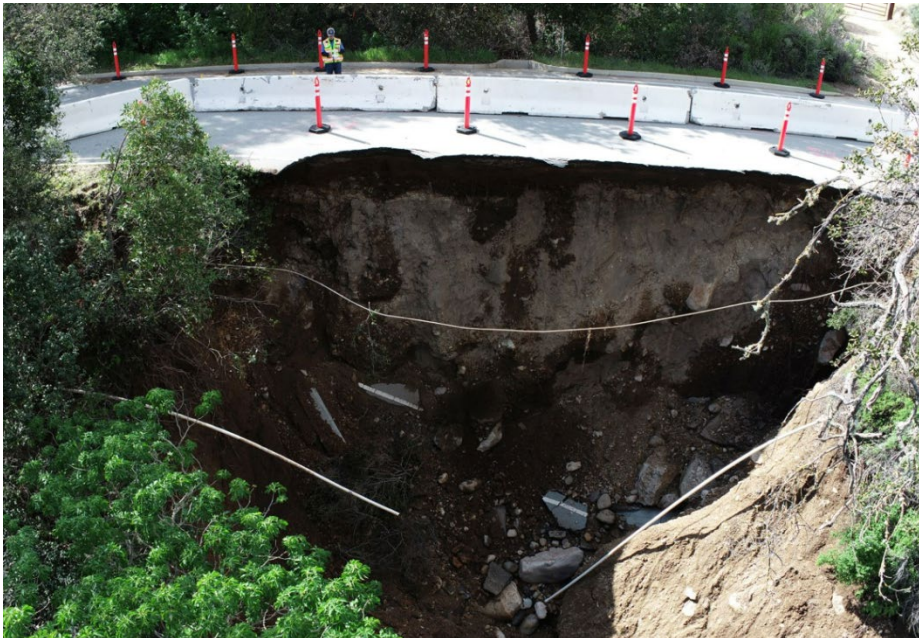
Road Scour and Failure
