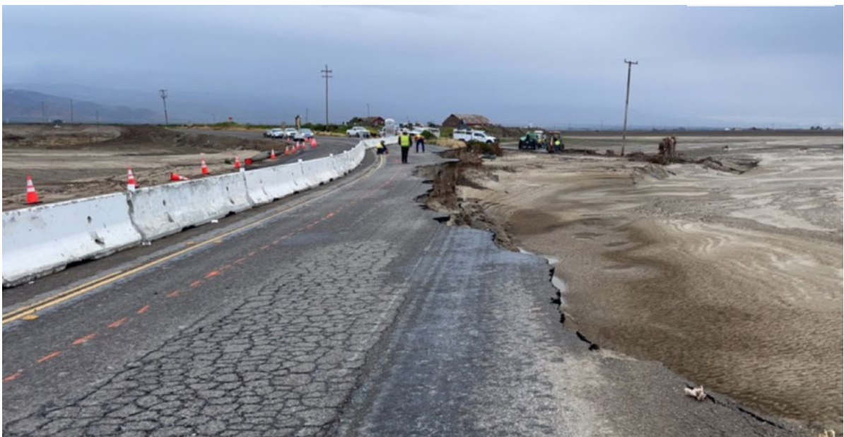
Road Scour and Failure
