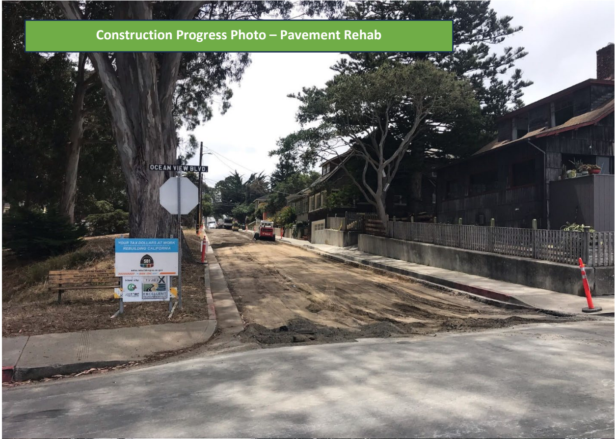
Construction Progress Photo – Pavement Rehab
