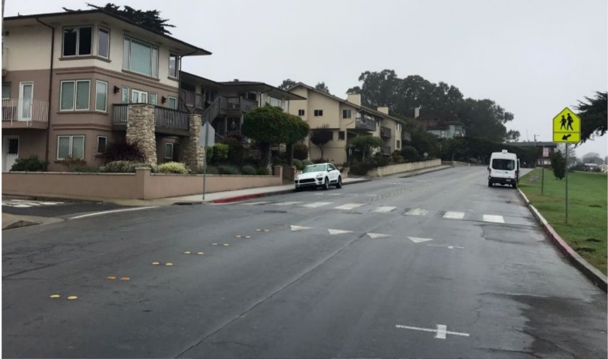
Before – Pedestrian & Road Improvements
