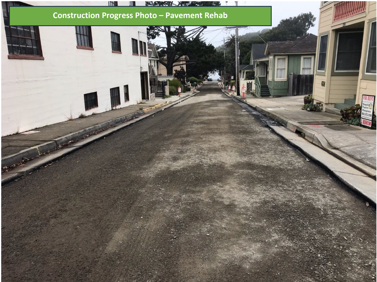
Construction Progress Photo – Pavement Rehab
