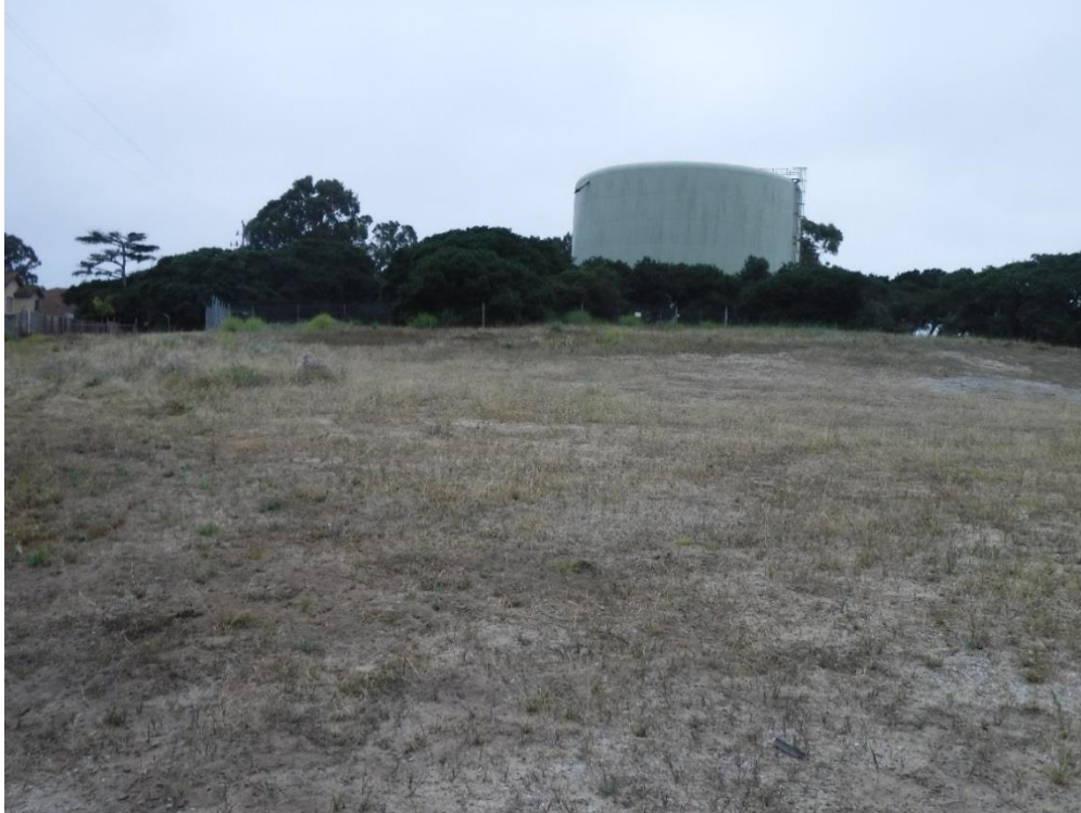
Photograph 33. 6.20.2019. Water tower located along the Northern Loop Trail segment with annual grassland in the foreground, facing west.
