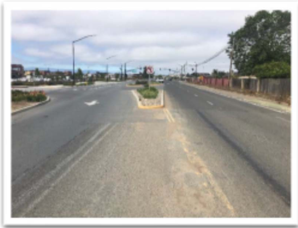
Before: San Juan Grade Road @ 120' N/O Northridge Drive facing South
