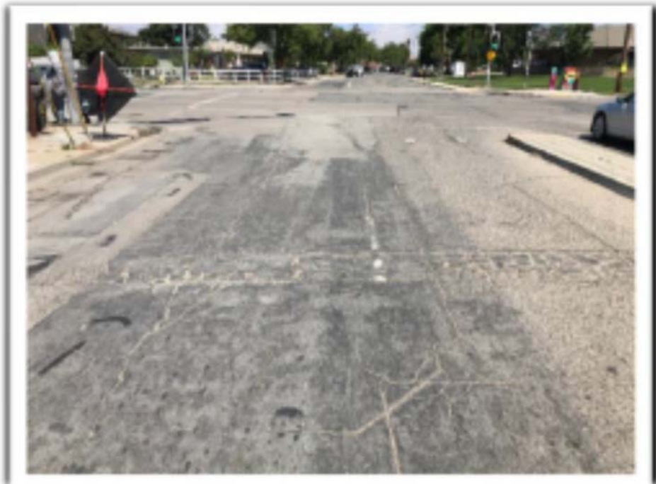
Before: Bardin Road @ Williams Road South Bound facing North intersection
