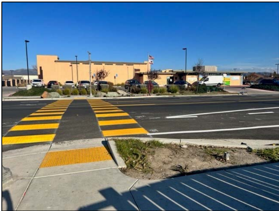
After: Bardin Road @ Toro Ave facing West
