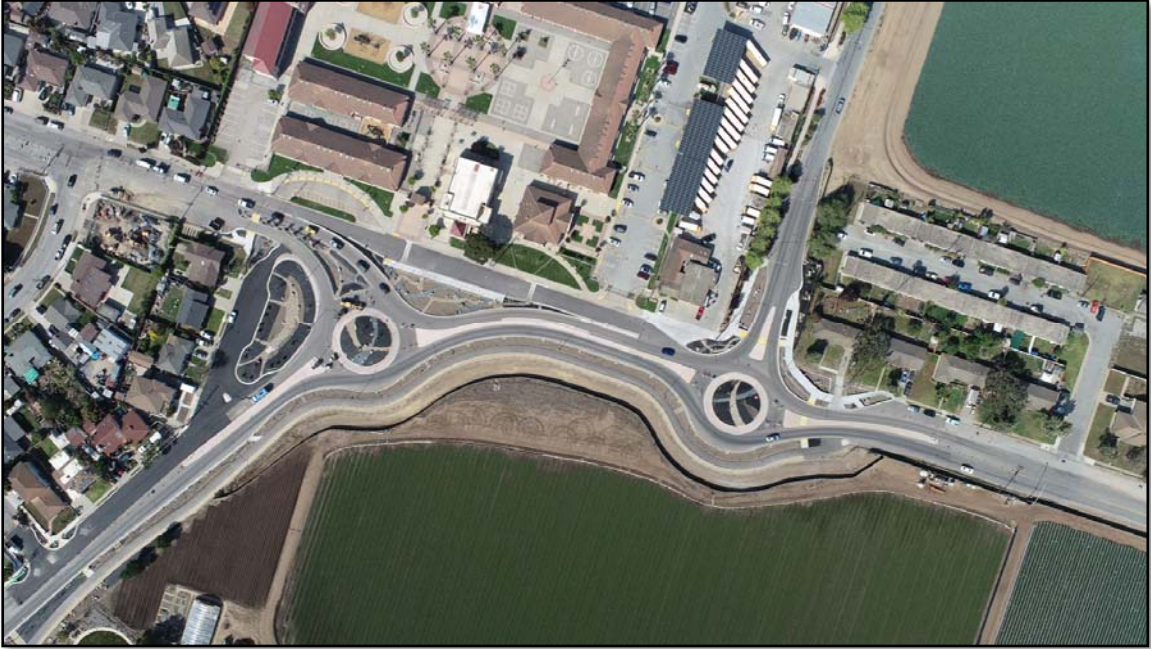
Aerial view of Bardin Road/Alisal St/Alisal Road intersection April 2022
