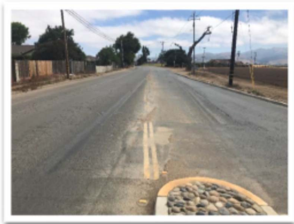
Before: San Juan Grade Road @ 120' N/O Northridge Drive facing North
