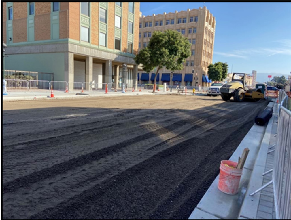
Construction Photo: Grading for New Roadway Pavement
