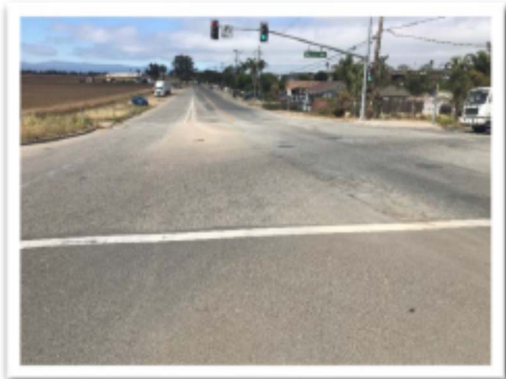
Before: San Juan Grade Road @ Russell Road facing South
