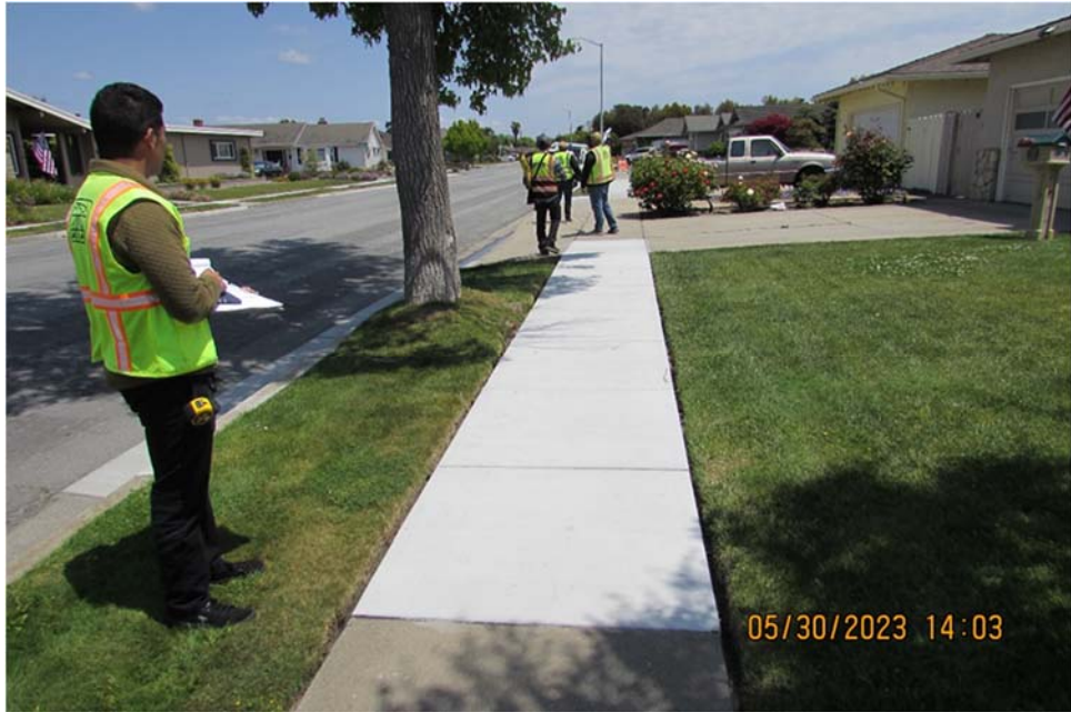
After photo of Palma Dr Citywide Sidewalk Repair Project
