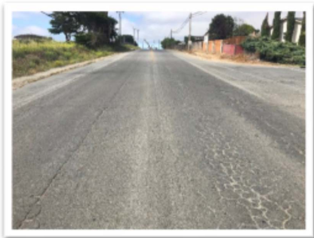
Before: San Juan Grade Road @ Van Buren Avenue facing South
