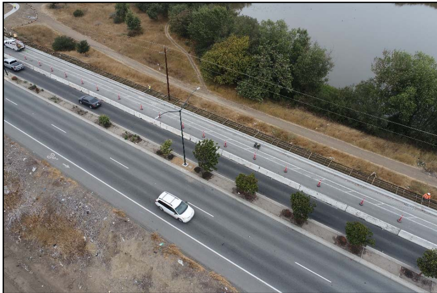
View of the pedestrian boardwalk under construction.
