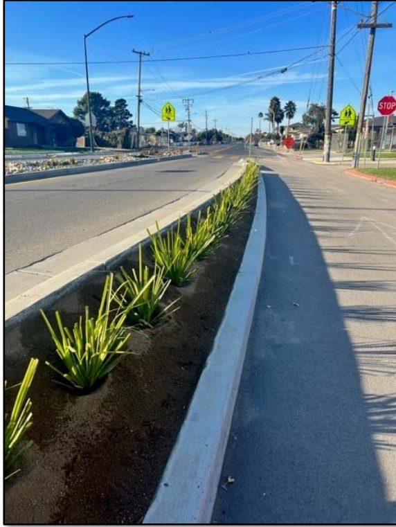
Bardin Road/Alisal St/Alisal Road intersection facing South
