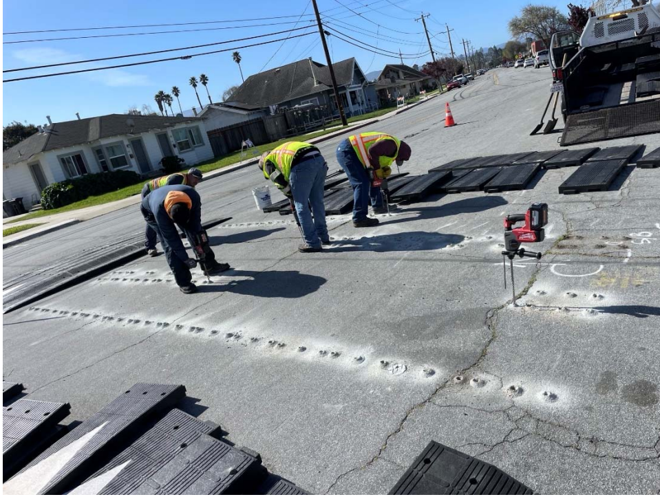
Construction Photo: Iverson Street traffic calming installation
