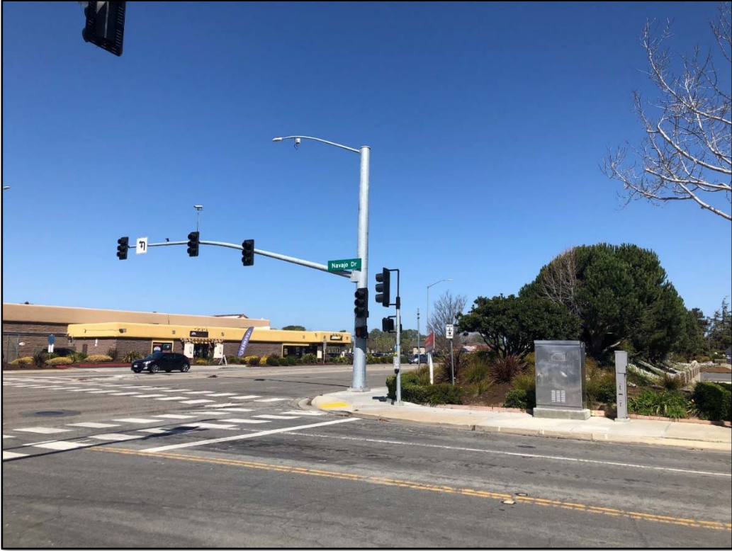
After Construction Photo: New signal facing northbound
