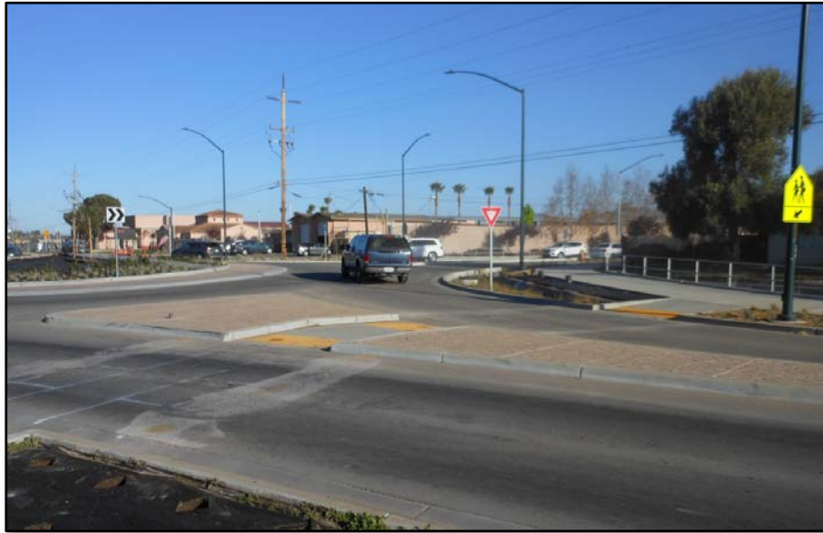
During Contrsution: Alisal Road near Sconberg Parkway
