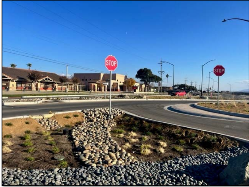
Bardin Road/Alisal St/Alisal Road intersection
