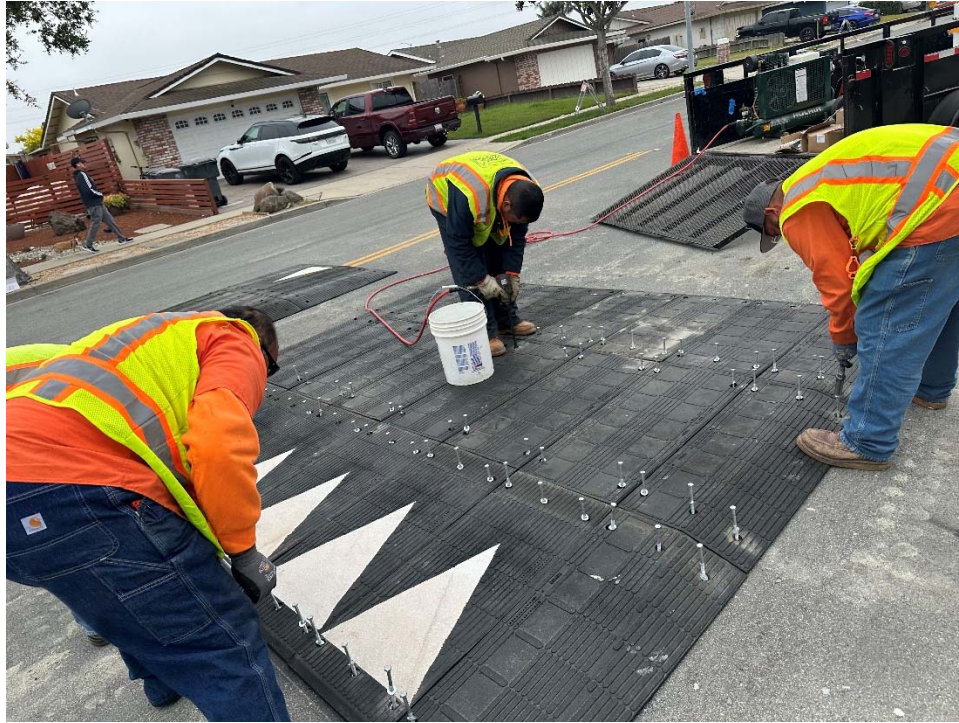
Construction Photo: Victor Street traffic calming installation
