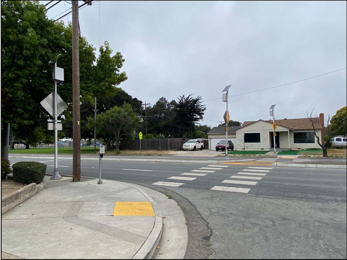
After Photo: W Laurel Drive at Parkside Street
