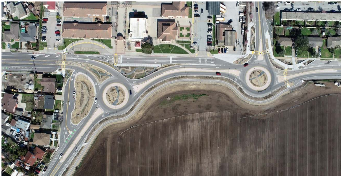
Aerial view of Bardin Road/Alisal St/Alisal Road intersection March 1, 2023
