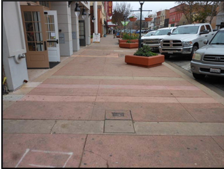
Before: 200 Block Sidewalk Facing South
