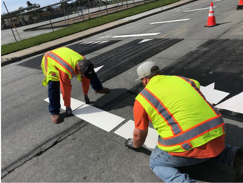
Construction Photo: West Acacia Street traffic calming installation
