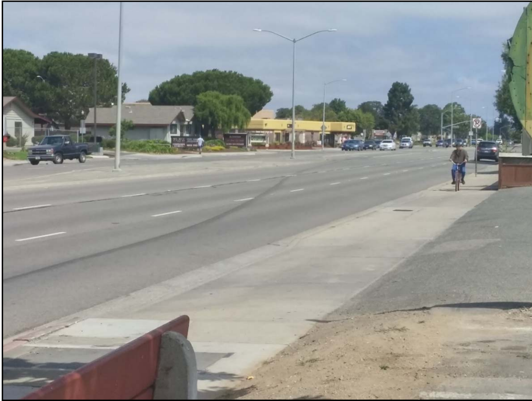
Before Photo: North Main Street Between Chaparral Street and Navajo Drive
