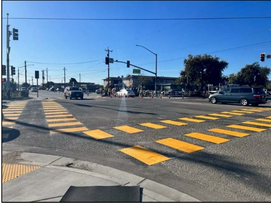
After: Bardin Road @ Williams Road intersection
