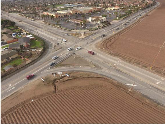
Existing Natividad/Boronda Intersection
