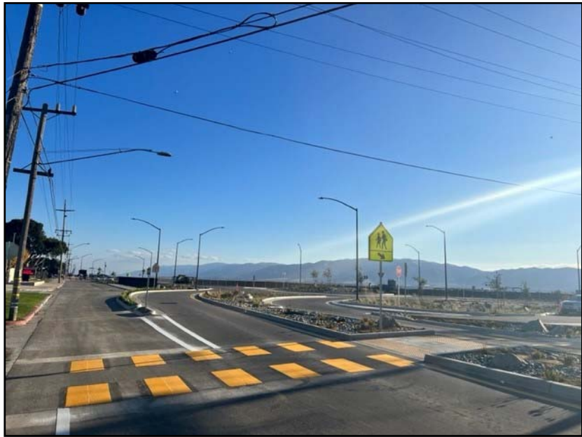
Bardin Road/Alisal St/Alisal Road intersection
