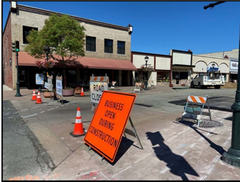
Main St at San Luis St: During Construction
