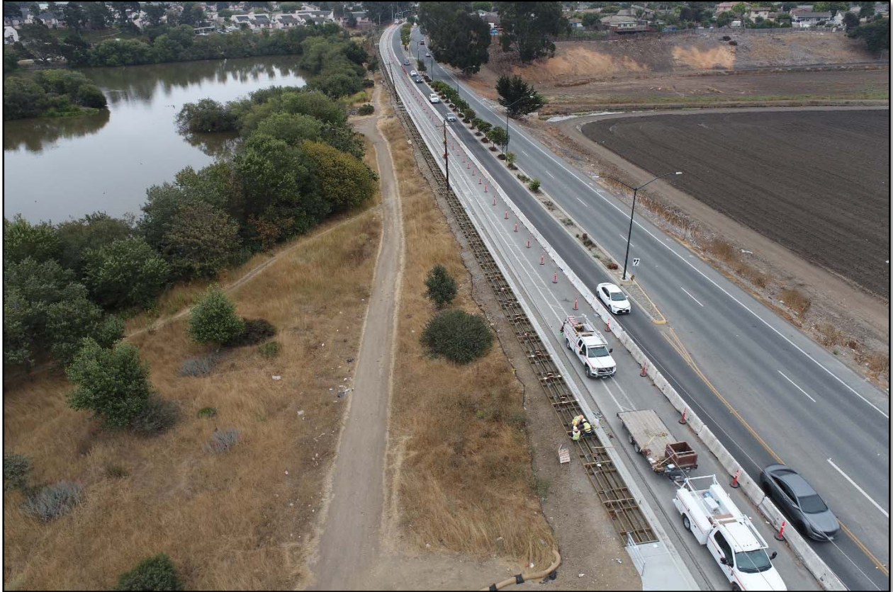
Laurel Boardwalk construction
