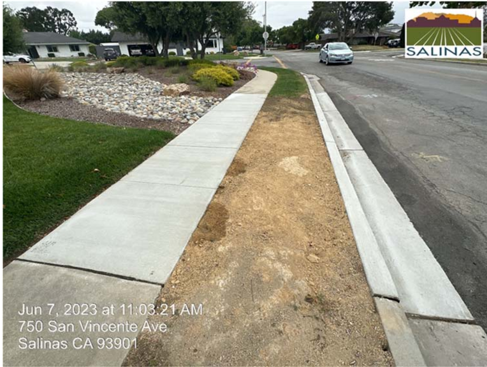
After photo of San Vicente Ave Citywide Sidewalk Repair Project
