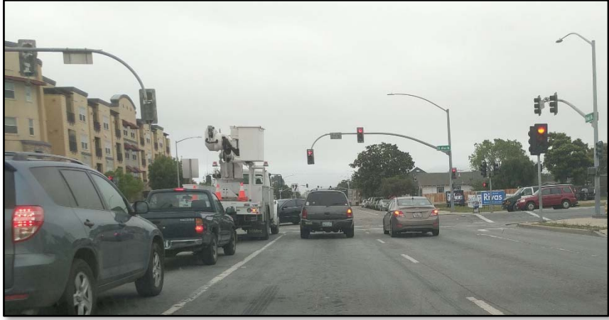
Existing conditions photo
