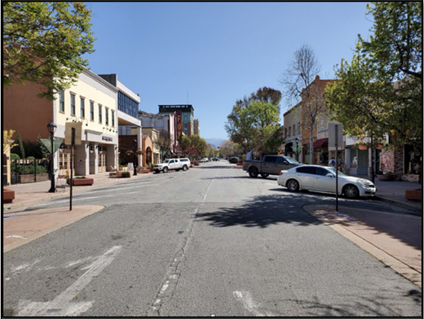
Before: 200 Block Facing South
