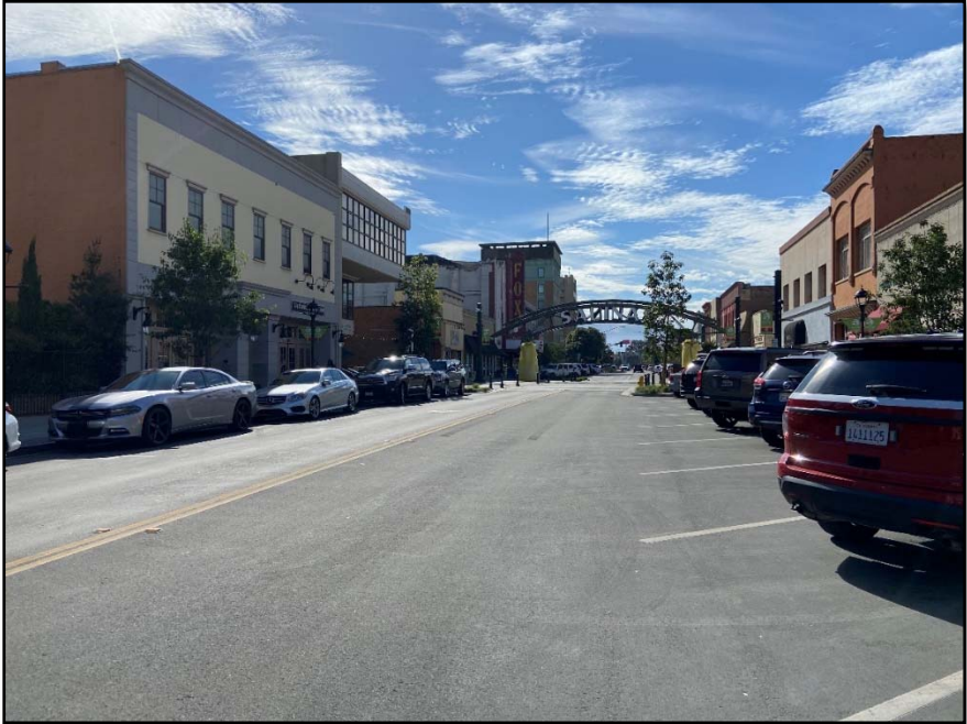
After: 200 Block Facing South
