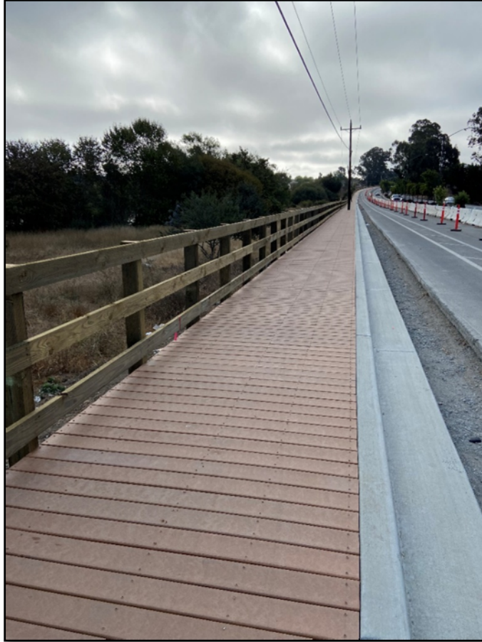
Pedestrian boardwalk completed.
