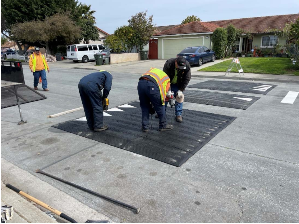
Construction Photo: Paseo Grande traffic calming installation
