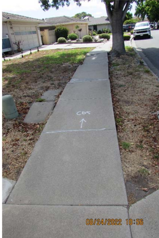
Before photo of Coleridge Dr. Citywide Sidewalk Repair Project
