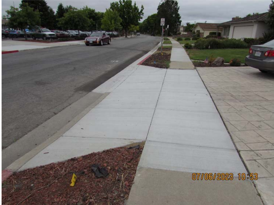
After photo of San Miguel Ave Citywide Sidewalk Repair Project
