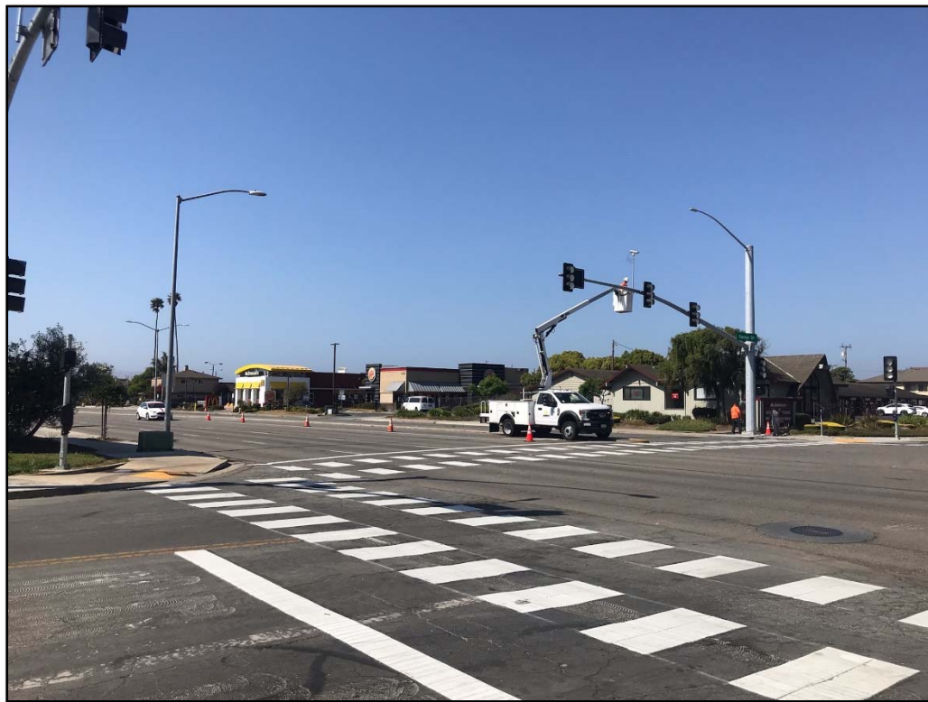
Construction Photo: Installing the Video Detection Cameras
