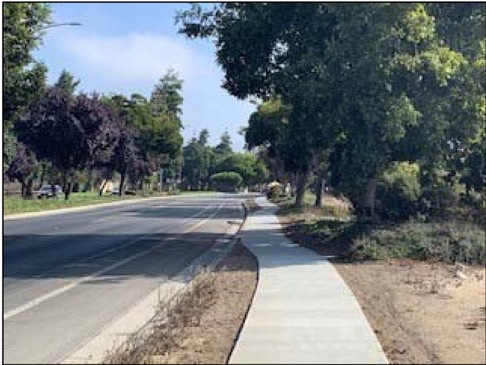
Constitution Blvd looking North – New sidewalk
