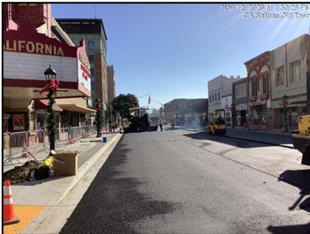
Construction Photo: 200 Block – Placing New Pavement
