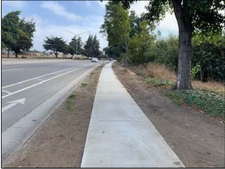
Constitution Blvd looking North – New sidewalk
