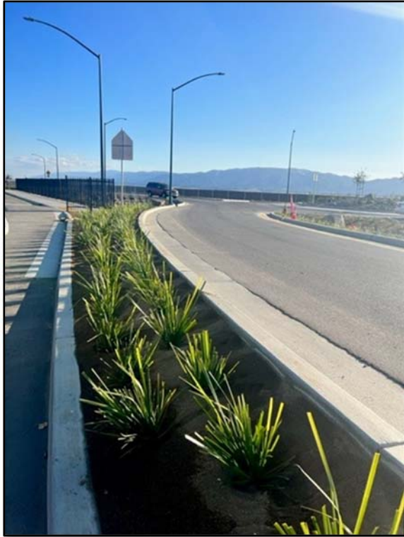
Bardin Road/Alisal St/Alisal Road intersection facing North
