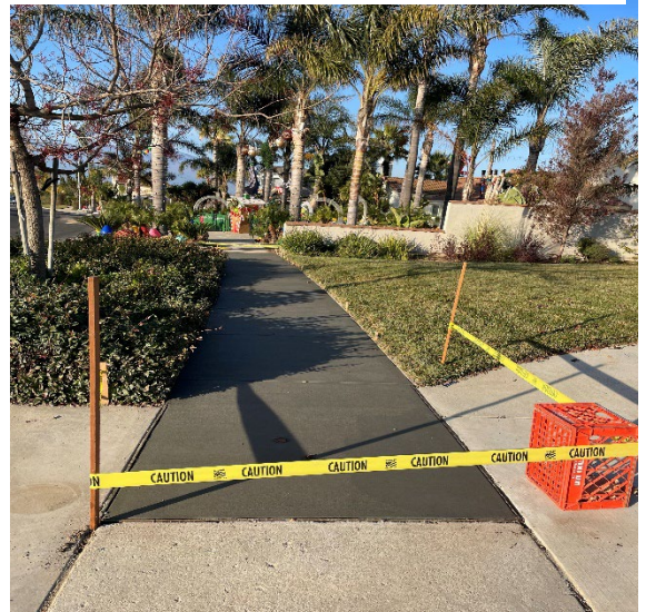
After Picture: 359 Blueridge Ct – New Concrete Panels.
