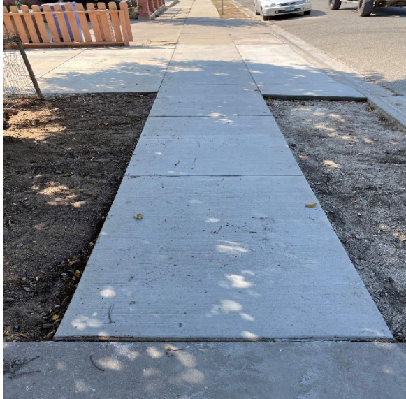
After Picture: 1200 Palm Ave – Sidewalk Closeup
