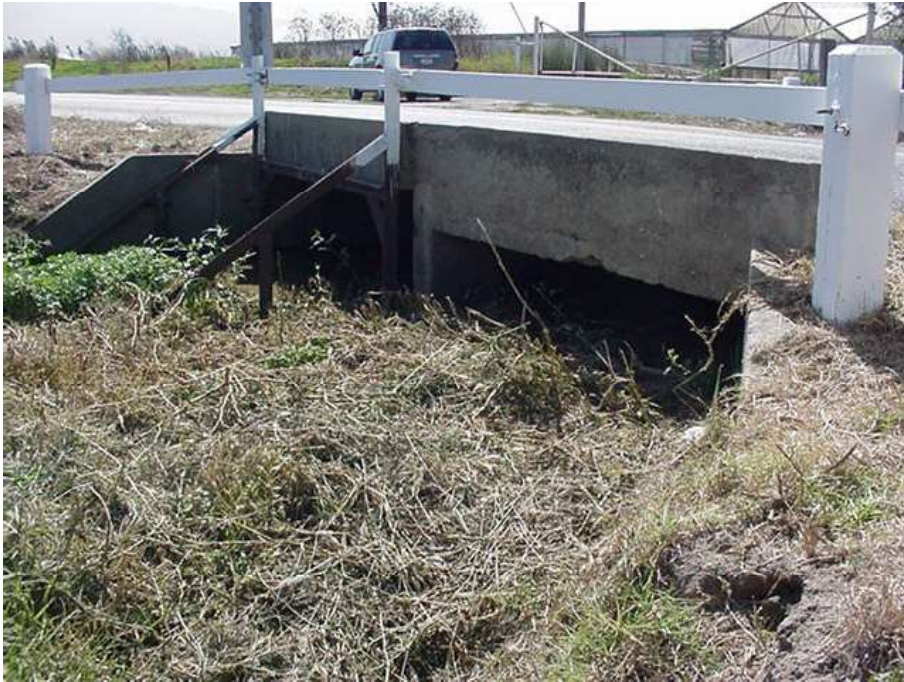
Previous bridge/box culvert
