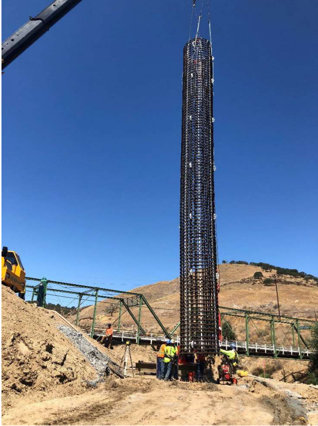
Setting of rebar cage for pier
