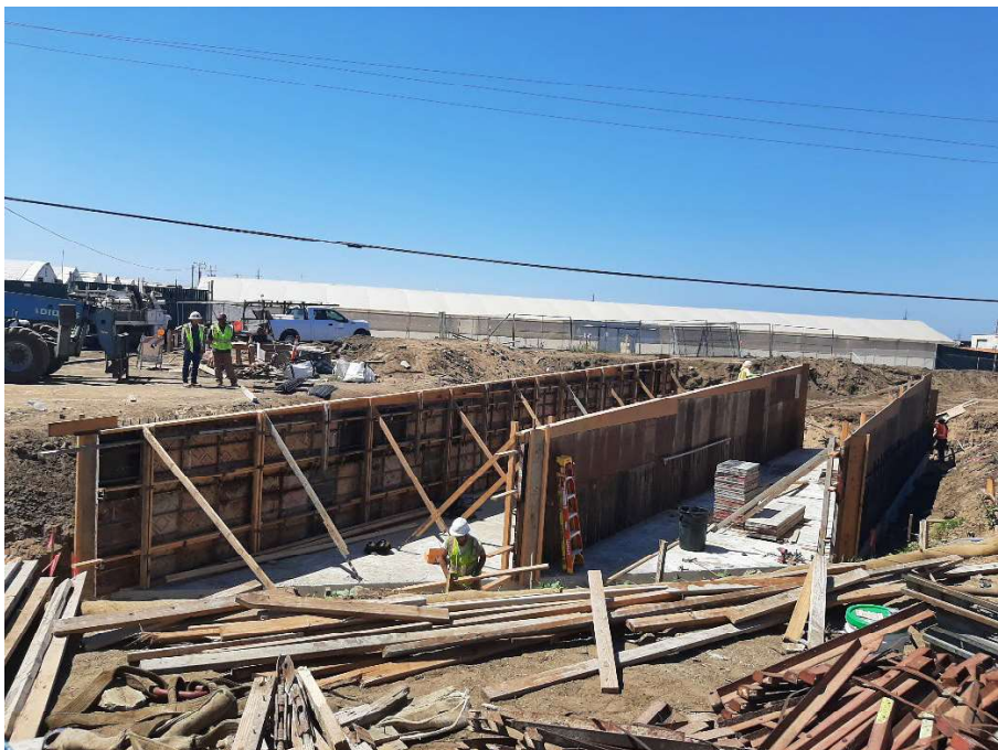
Form work for new bridge
