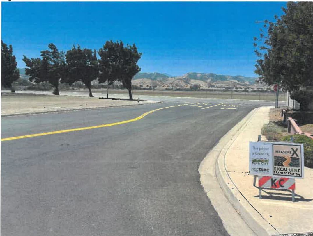
Figure 2 Willow Street at San Antonio Drive - After
