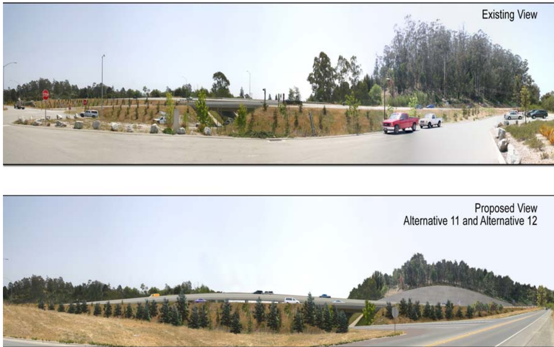
Figure 2-7 Existing and proposed view from Prunedale North Road, near the park and ride lot and the existing U.S. Route 101/State Route 156 interchange looking south
