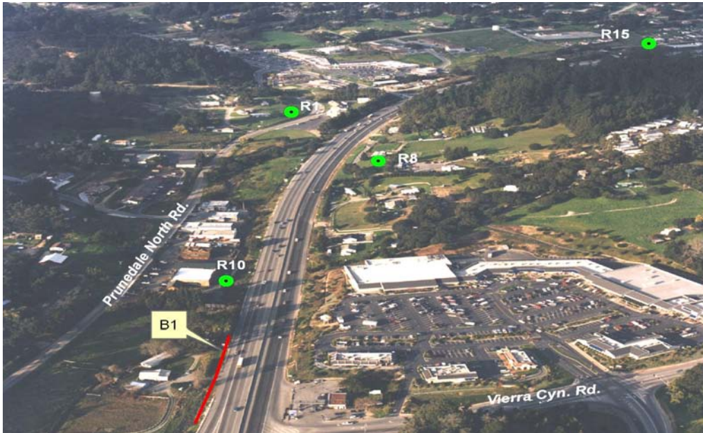
Figure 2-13 Receivers 1, 8, 10 and 15 and Barrier 1 near U.S. Route 101, north of Vierra Canyon Road
