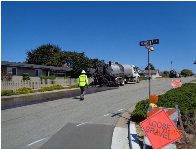
Figure 4 - Tack Coating (Step 1)
