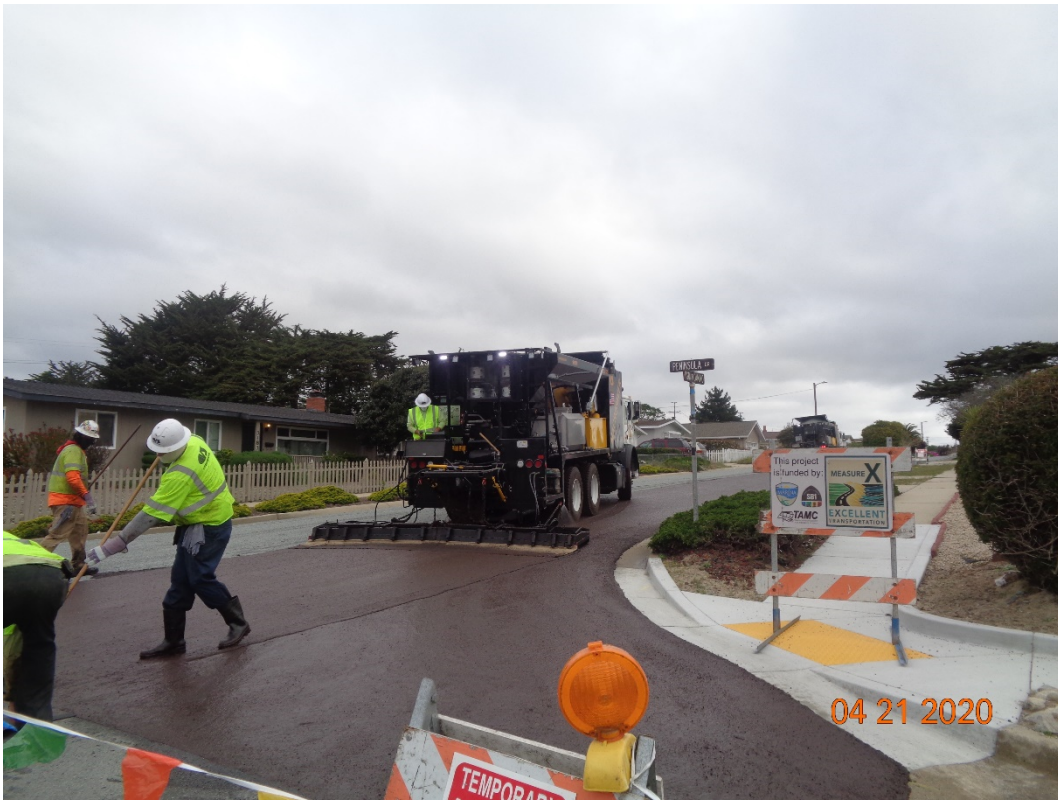
Figure 6 - Final Slurry Coating (Step 3)
