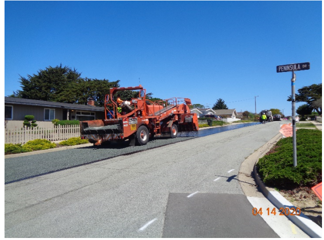
Figure 5 - Spreading Chip Aggregate (Step 2)
