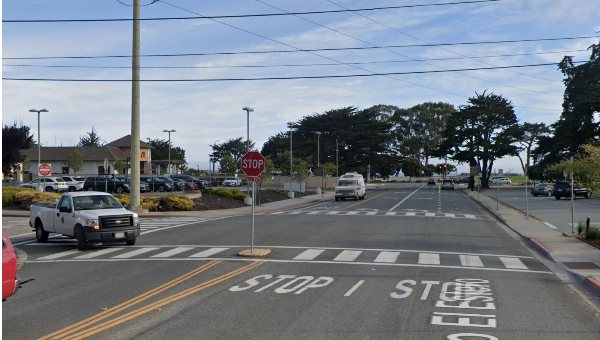
Camino El Estero at Franklin St, Before Post Alerts 2021
