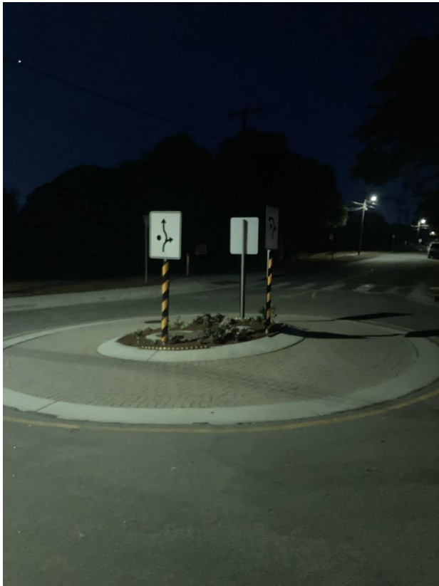
Virgin Avenue Traffic Circle at Grant, After Post Alerts (Nighttime) 2023
