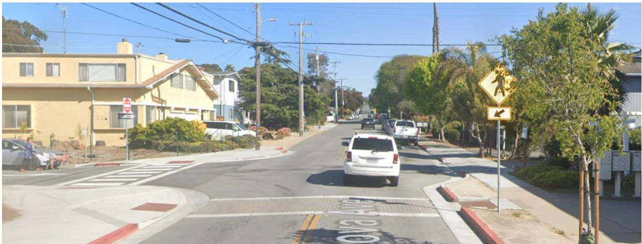
Before Rectangular Rapid Flashing Beacon Installed, 2022
