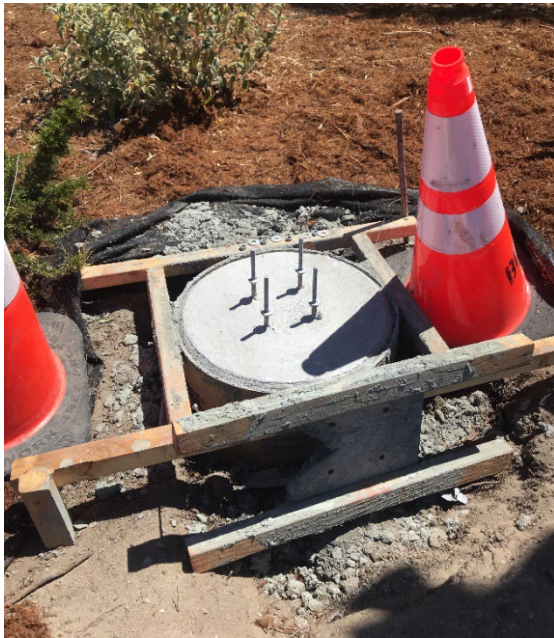
Wayfinding sign foundation construction
