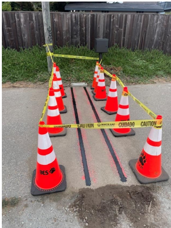
Installation of the Bicycle Counters at Location 2, 2023
