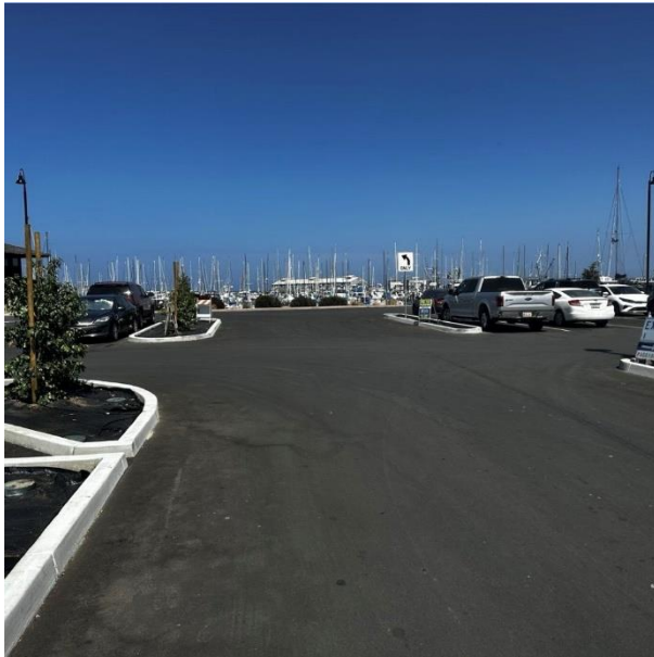
Marina Parking Lot Improvements, 2023
