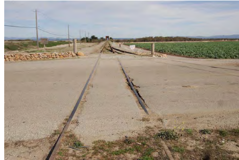
North Dole Grade Crossing (MP 113.80)
