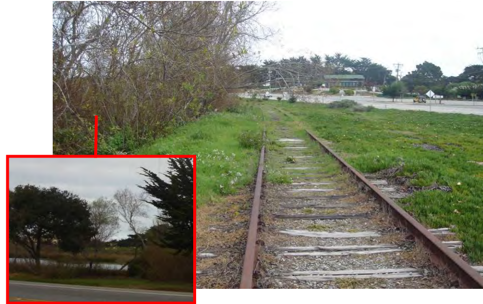
Figure 9-66 Track at Reservation Road Looking North
