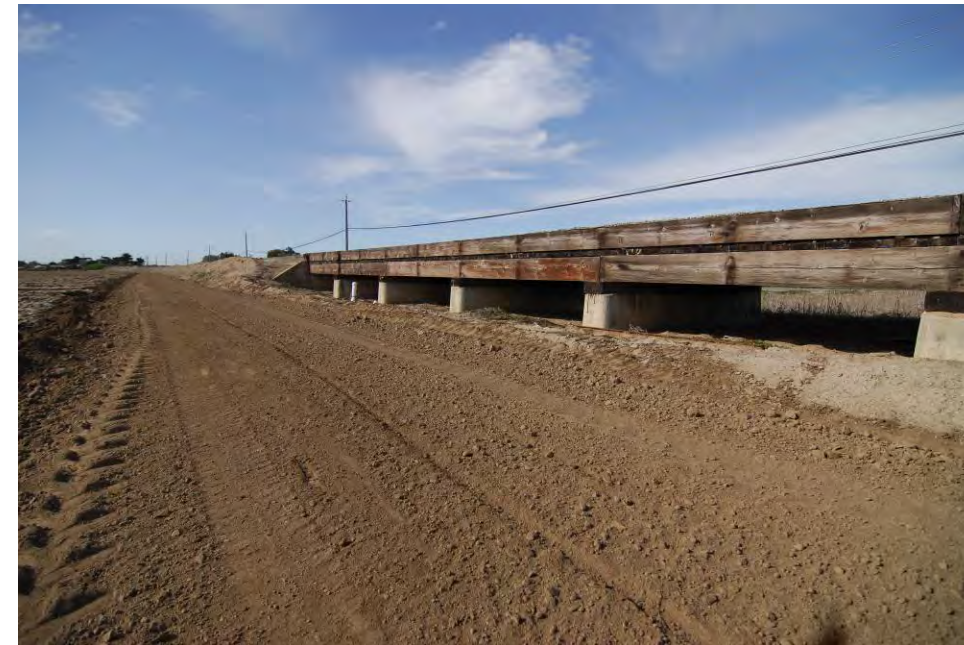
Floodplain Equalizer Timber Trestle Bridge Foundation (MP 113.04)
