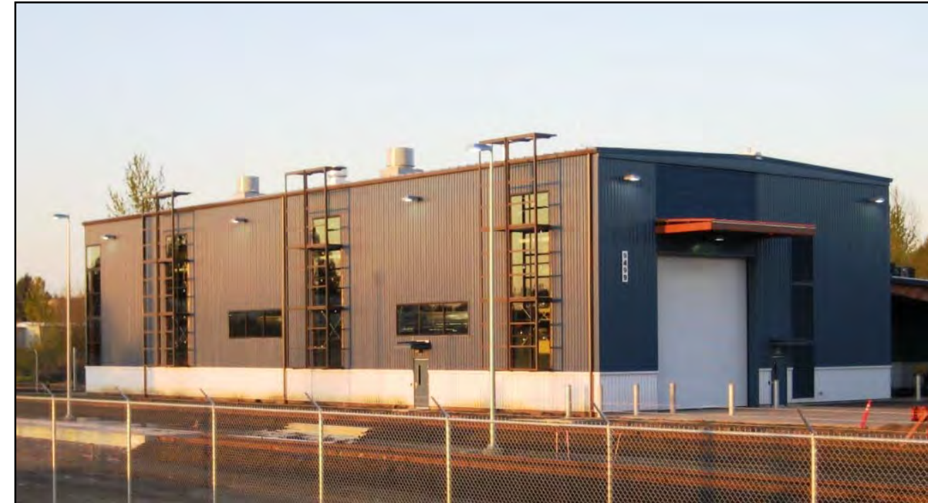
Figure 6-1 Maintenance Facility Servicing a Diesel Multiple Unit Vehicle Fleet (Westside Express Service, Tri-County Metropolitan Transportation District of Oregon)
