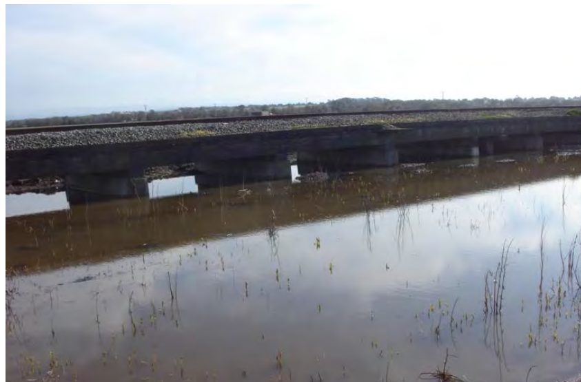
Figure 9-47 Floodplain Equalizer Trestle Bridge at MP 112.8
