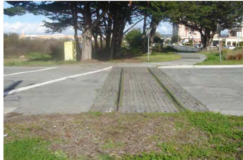
Figure 9-84 Grade Crossing at Roberts Avenue
