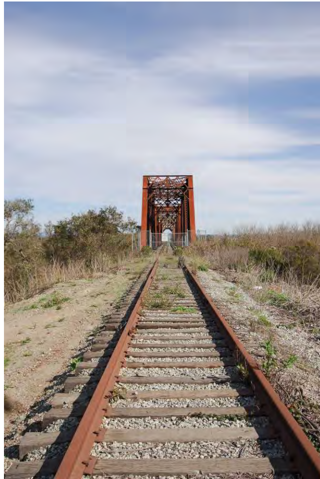
Closed Salinas River Bridge and Track (MP 113.50)
