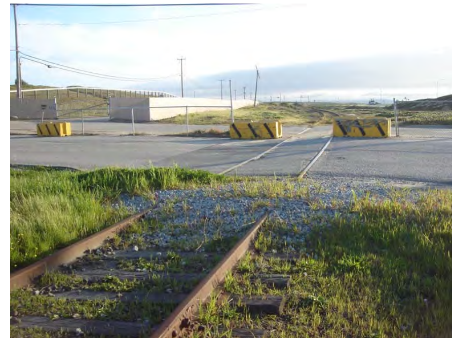
Figure 9-57 South Dole Grade Crossing
