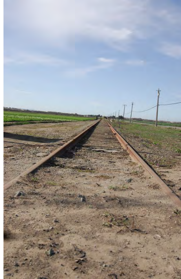
Condition of Trackwork near Nashua Road (MP 112.50)
