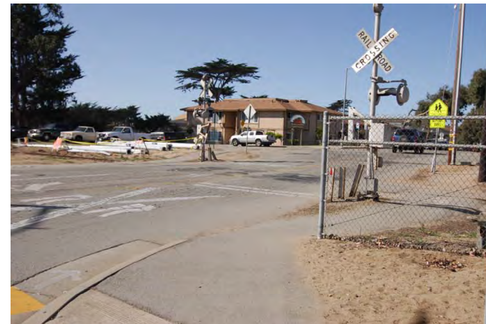
Westerly View at Palm Avenue Grade Crossing (MP 117.30)
