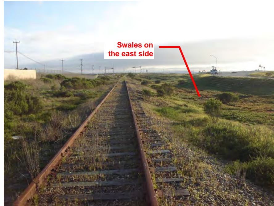
Figure 9-58 Drainage South of Lapis Road
