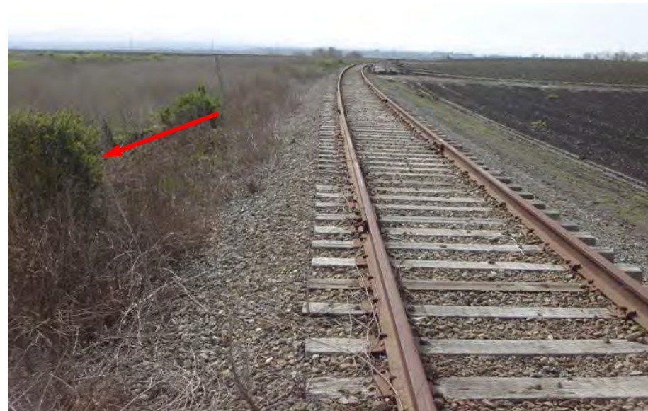
Figure 9-31 Rail South of Merritt Street Looking South
