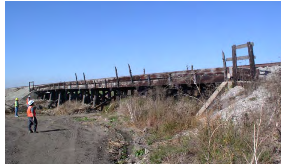
Southwesterly View of Trembladero Slough Bridge (MP 111.05)
