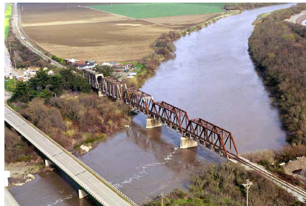
M.P. 113.46—Salinas River Bridge, 715-foot Steel Through Truss Bridge
