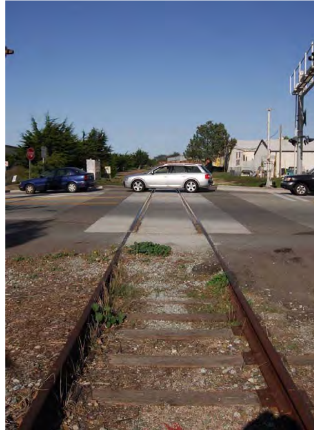
Northerly View of Grade Crossing at Tioga Avenue (MP 122.80)
