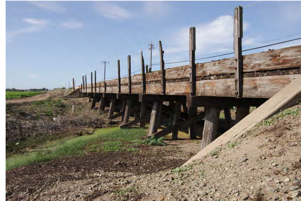
Drainage Channel Bridge Trestles (MP 112.54)
