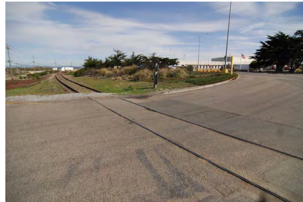
South Dole/Ranch Grade Crossing (MP 114.07)
