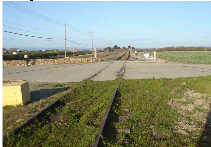
Figure 9-55 North Dole Grade Crossing
