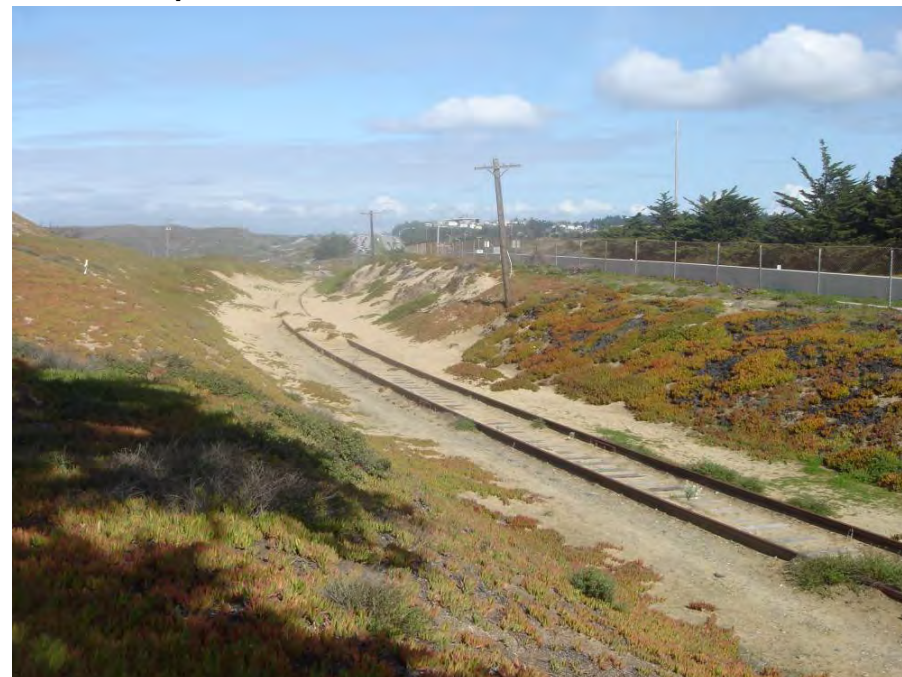
Figure 9-74 Rail at State Route 1 Overpass
