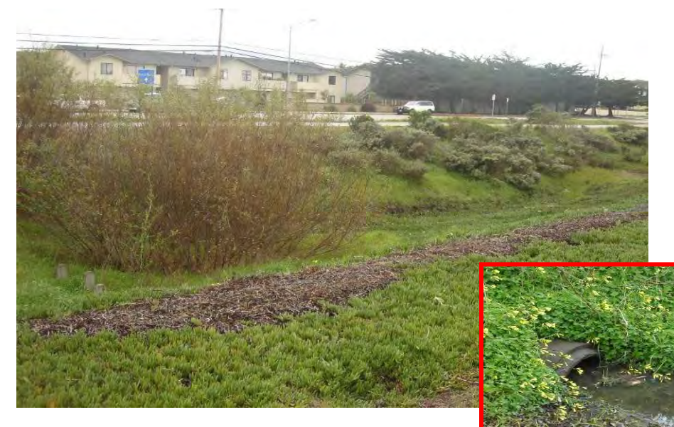
Figure 9-64 Swale at the Southeast of Marina Green and Rail with a Culvert
