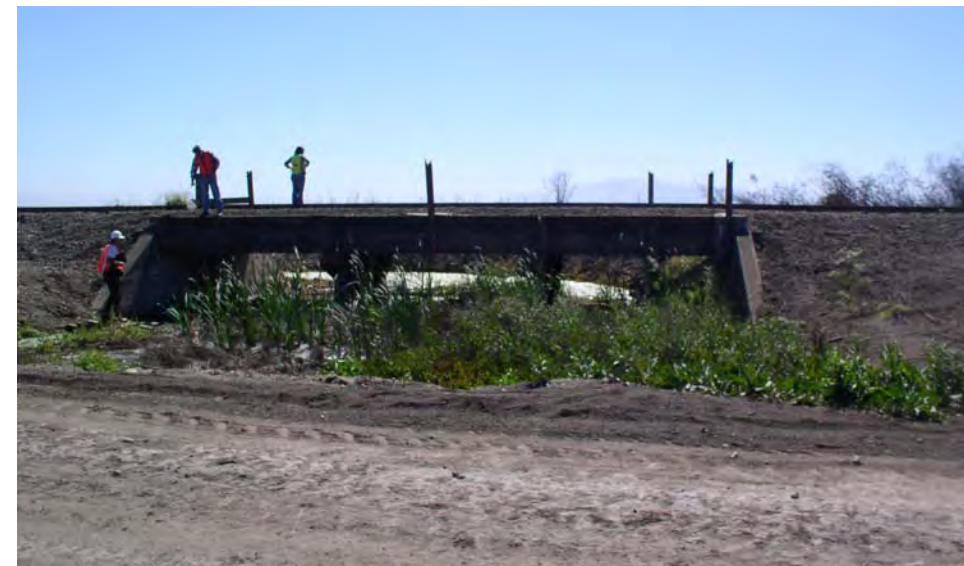
Alisal Slough Bridge prior to Reconstruction (MP 111.93)
