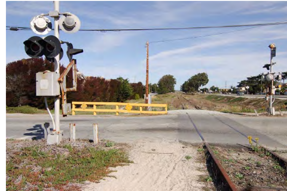
Northerly View at Beach Road Grade Crossing (MP 116.50)
