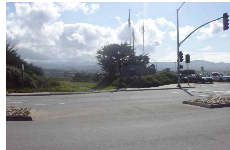
Figure 9-75 Monterey Road Grade Crossing (610+00)
