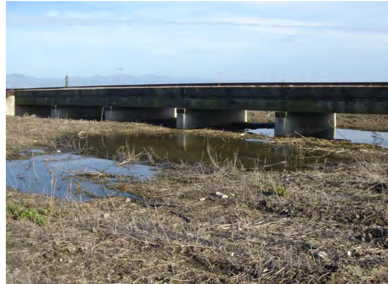
Figure 9-50 Floodplain Equalizer Timber Trestle Bridge at MP 113.04
