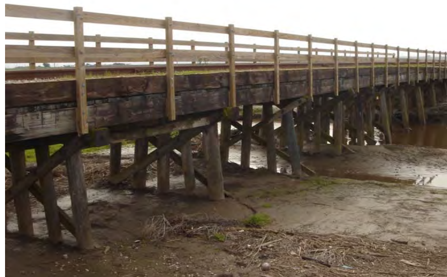
Figure 9-34 Bridge at Tembladero Creek
