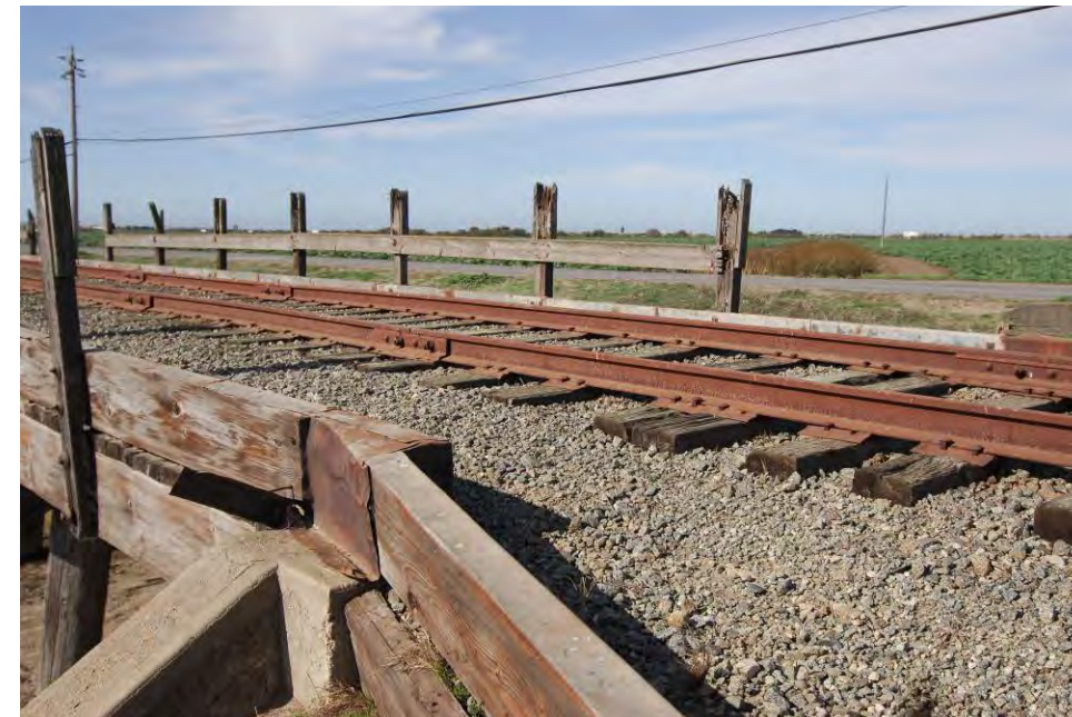
Drainage Channel Bridge Trackwork and Structure (MP 112.54)
