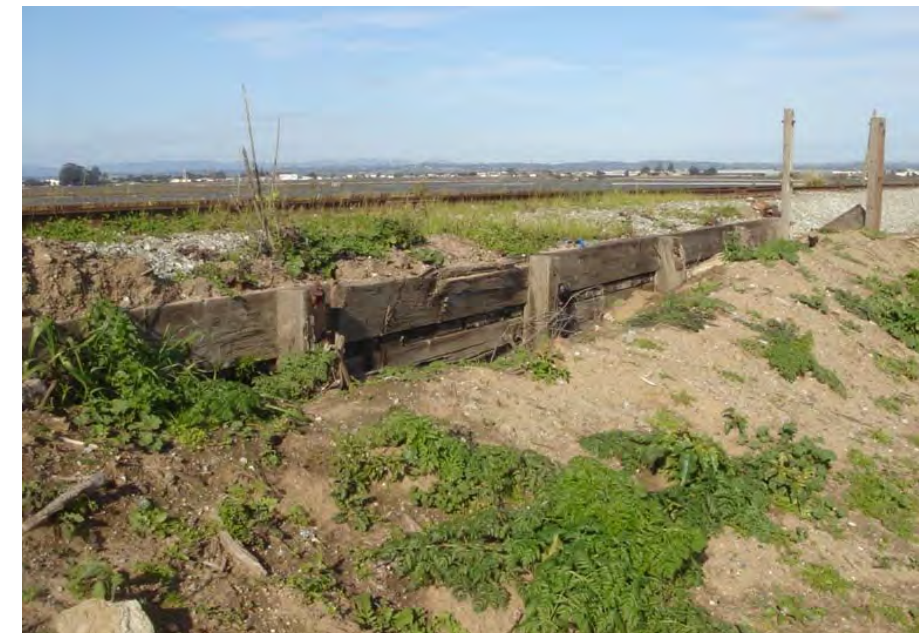
Figure 9-37 Alisal Earth Embankment at MP 111.93
