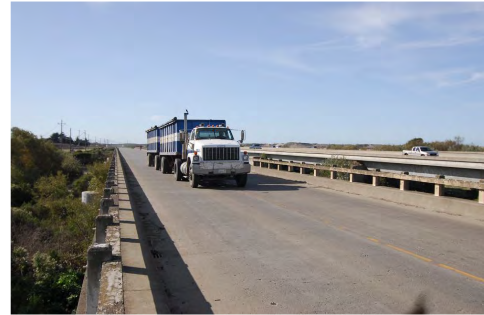
Salinas River Bridge Roadway
