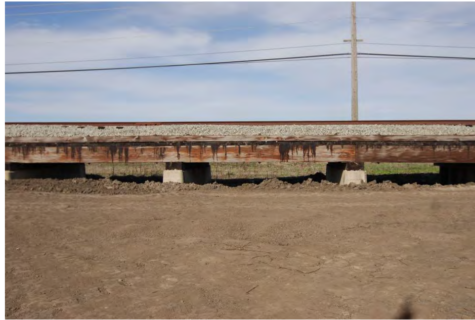
Floodplain Equalizer Trestle Bridge (MP 112.8)
