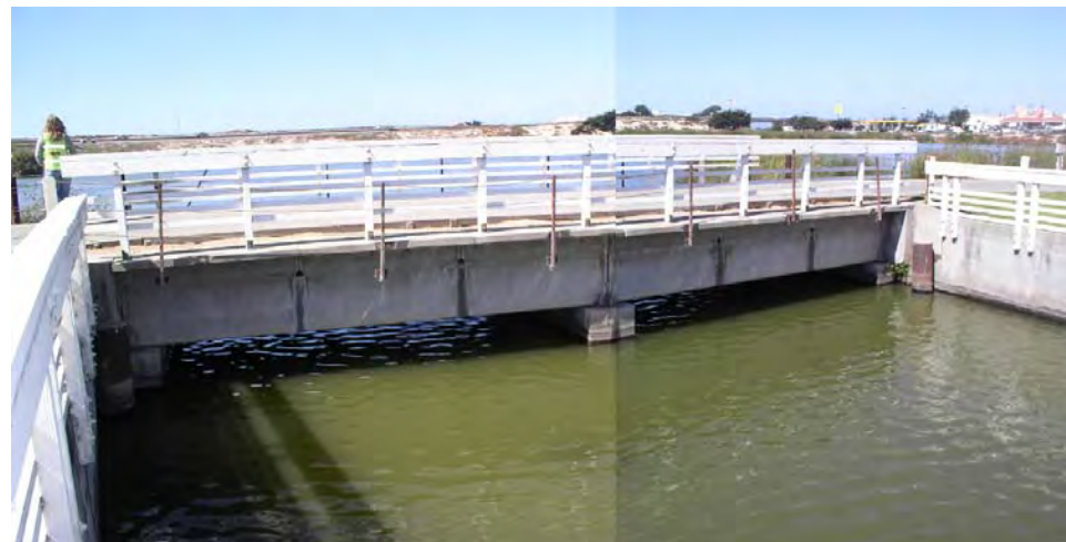
Roberts Lake Bridge (MP 123.80)
