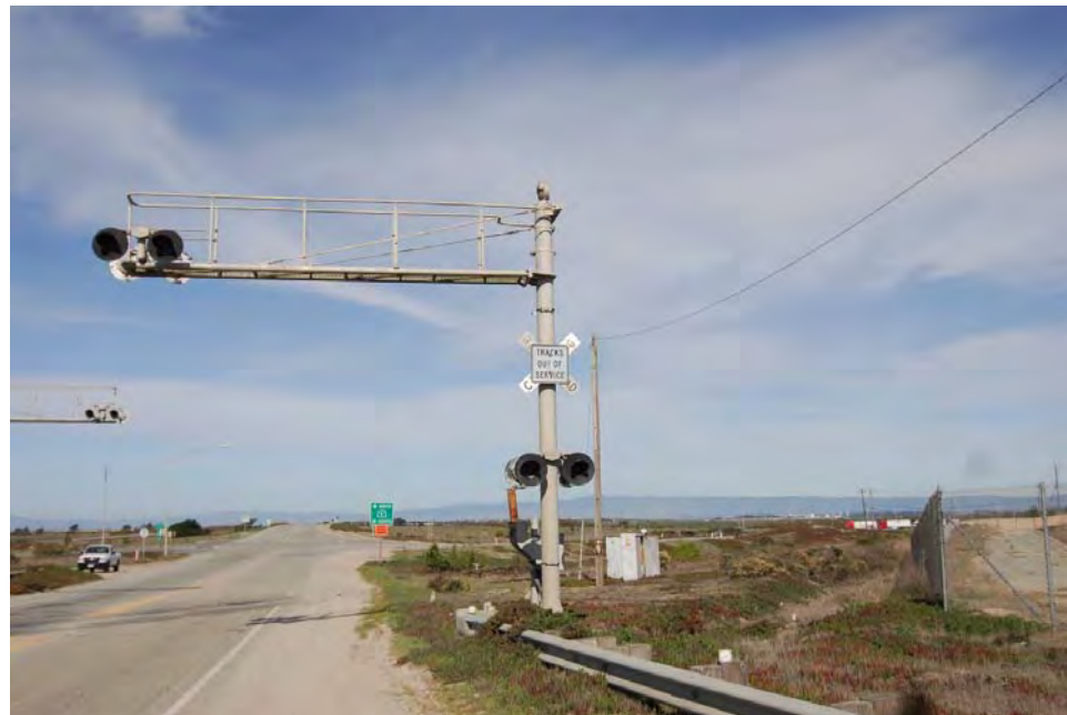
Grade Crossing at Del Monte Boulevard (MP 114.30)
