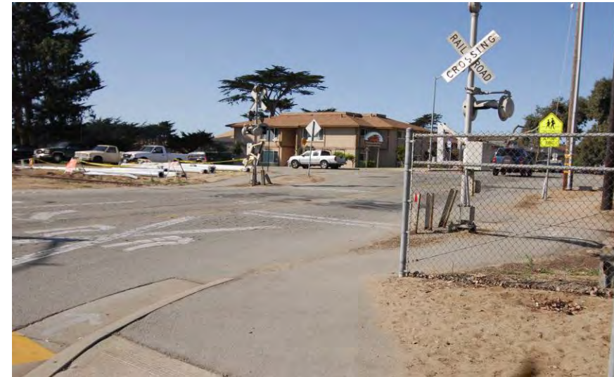
Figure 9-68 Westerly View at Palm Avenue Grade Crossing
