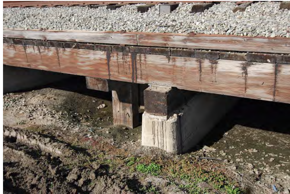
Floodplain Equalizer Bridge Foundation (MP 112.8)
