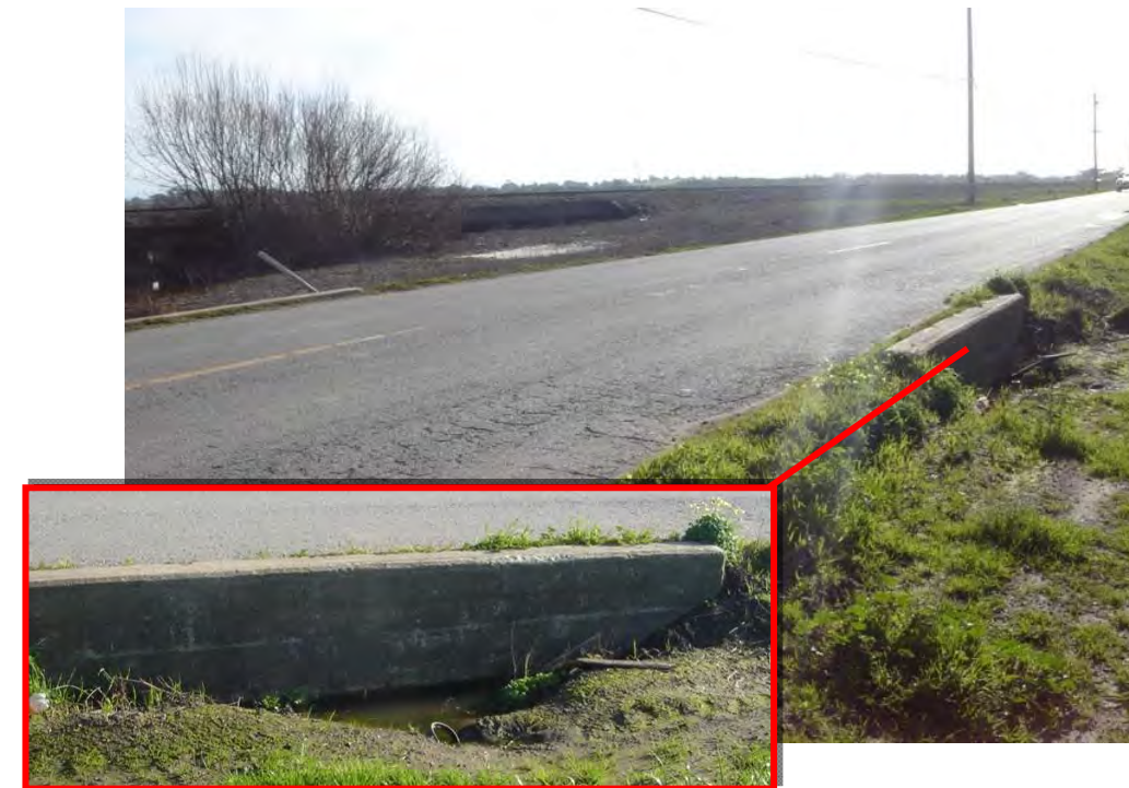
Figure 9-49 Culvert at Monte Road
