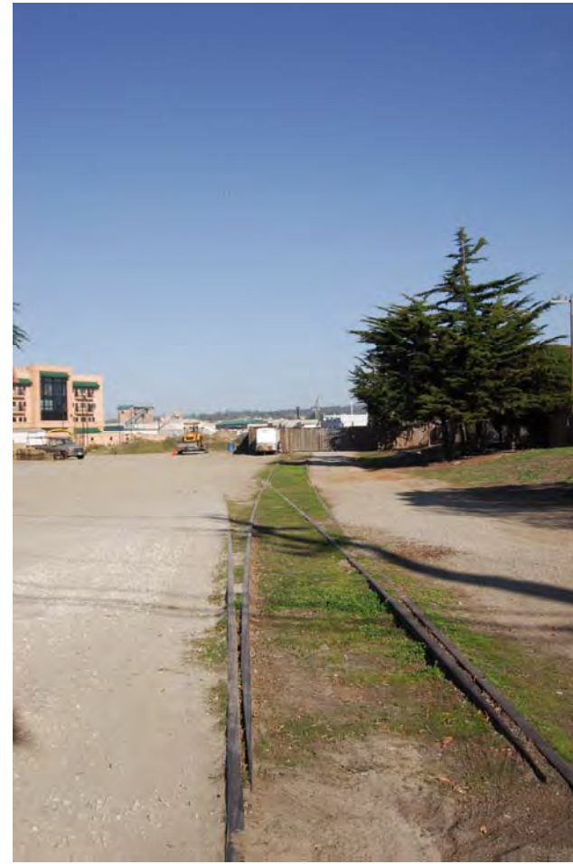
Easterly View of Railroad Right-of-Way at Contra Costa Street (MP 123.36)
