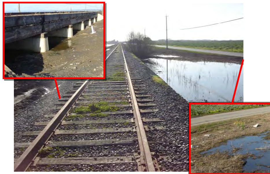
Figure 9-51 Ponding at the Floodplain Equalizer at MP 113.04
