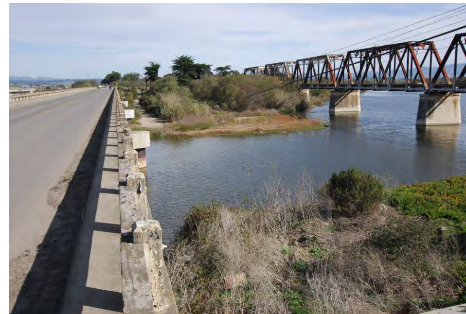
Existing and Closed Salinas River Bridges (MP 113.50)
