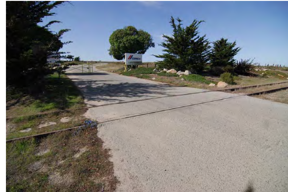
Cemex Grade Crossing off Lapis Road (MP 115.04)
