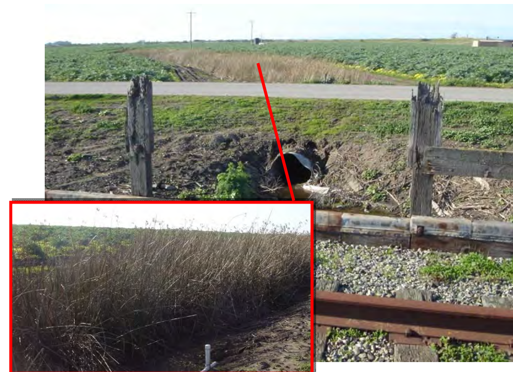
Figure 9-45 Culvert at MP 112.54
