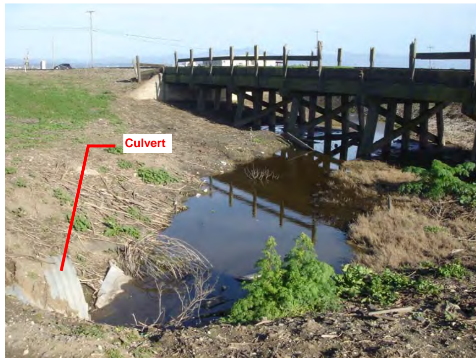
Figure 9-43 Bridge at MP 112.54
