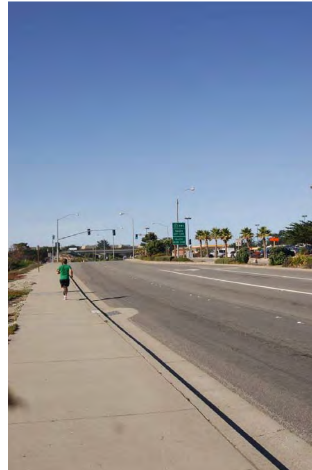
Northerly View near Canyon del Rey Boulevard (MP 123.60)
